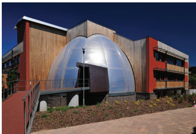
Figure 1. William Smith Building, British Geological Survey (BGS), Nottinghamshire. This building achieved a BREEAM excellent rating. BGS©NERC.
