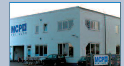
Head-Quarters & Demo-Center, Lübeck · Germany
