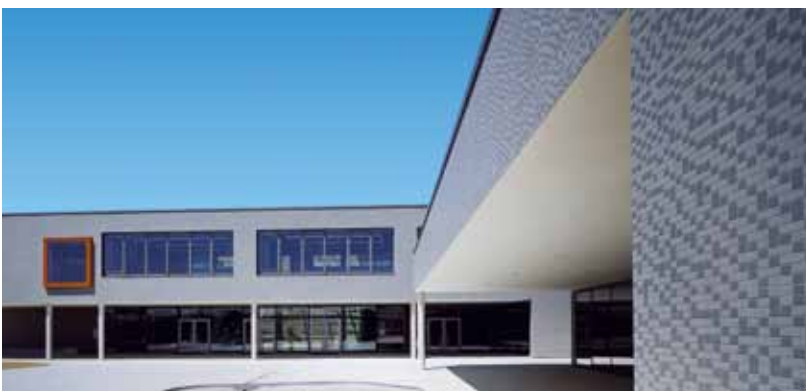
Elementary school, Erding/Germany Architectural firm: Dinkel, Persch/Stefan Dinkel, Munich/Germany StoVentec with ceramics
