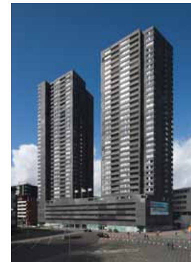
10 HOGHE HEREN (2005) Architect: Wiel Arets Architects Address: Gedempte Zalmhaven 179
