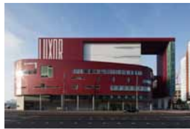
22 NIEUWE LUXOR THEATER (2001) Architect: Bolles & Wilson Address: Posthumalaan 1
