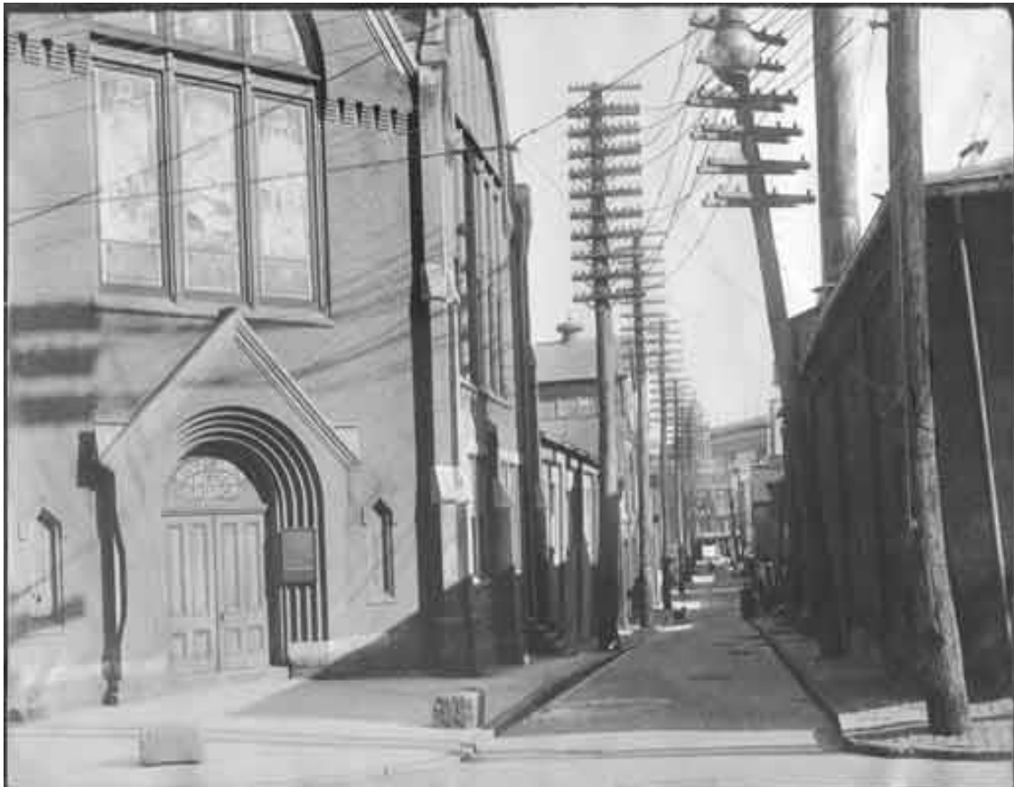
Wesley Union AME Zion Church in 1910, at the corner of South Street and Tanner's Alley
