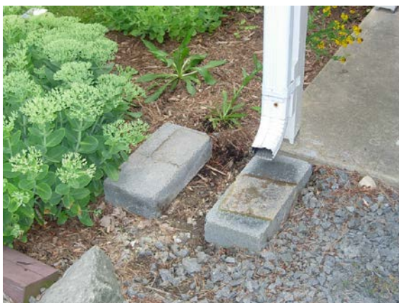
Concrete block can be used as platform
