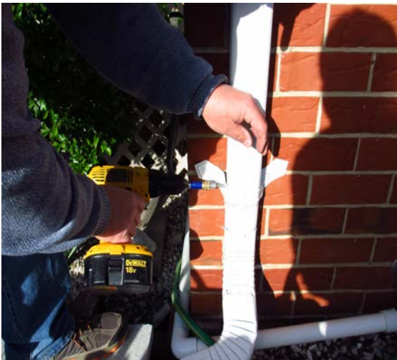
Reattach downspout straps
