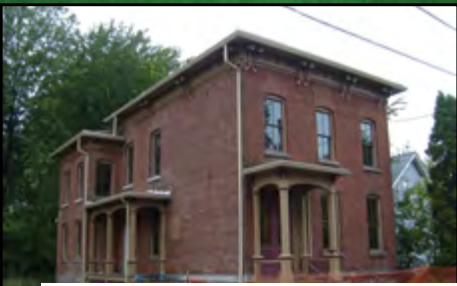
504 Niagara Street An exterior renovation to historic standards
