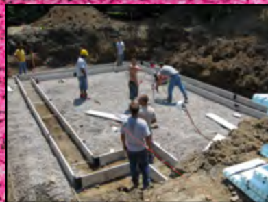
Opportunity HeadQuarters preparing an ICF foundation
