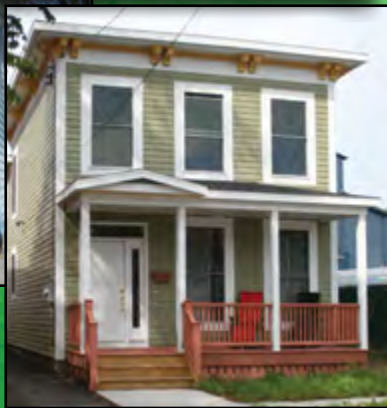
318 Marcellus Street - Full Rehab
