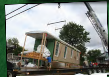
626 Gifford Street being delivered - a visitable, modular home
