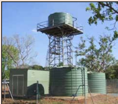
Water is pumped from the billabong (left) and treated in water treatment plant at Patonga Homestead (right). This system is now powered by the Bushlight automatic hybrid system.
