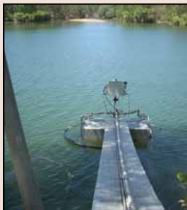
Water is pumped from the billabong (left) and treated in water treatment plant at Patonga Homestead (right). This system is now powered by the Bushlight automatic hybrid system.
