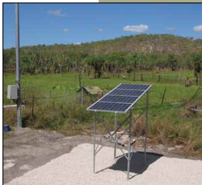
The new solar bore at Spring Peak which replaced a diesel run bore
