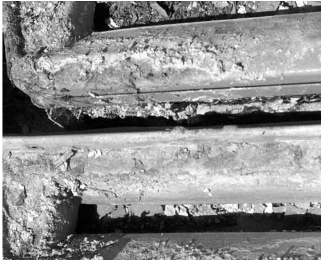
THE BUILD-UP OF CALCIUM (LEFT) BLOCKS WATER FLOW TO THE PADS. ONCE THE FILTER BASKET IS BLOCKED LIKE THE ONE ABOVE, NOT ENOUGH WATER WILL GET THROUGH TO THE PUMP. CLEAN BY SCRUBBING IT WITH A STIFF BRUSH AND WATER.
