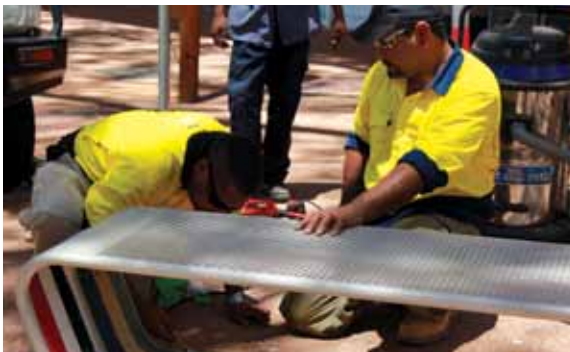
CAT Enterprise staff installing bench seats in Alice Springs mall.
