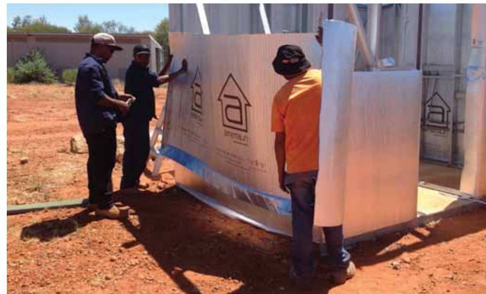
Phil Coombes, Roland Dann and Shaun Cummings constructing the abluition block.
