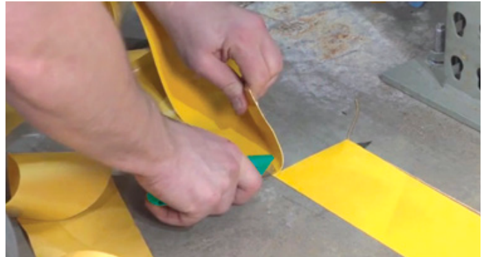
A razor blade may be used to cut out the damaged section of the floor tape.
