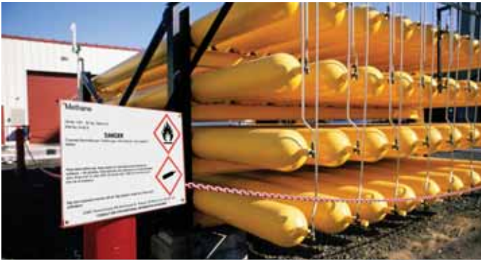
Large-format signs using the GHS style can also be used to mark storage areas.
