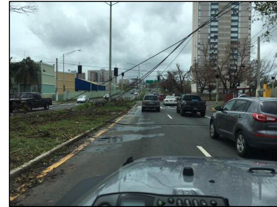
Downed power lines in Puerto Rico following Hurricane Maria in 2017.
