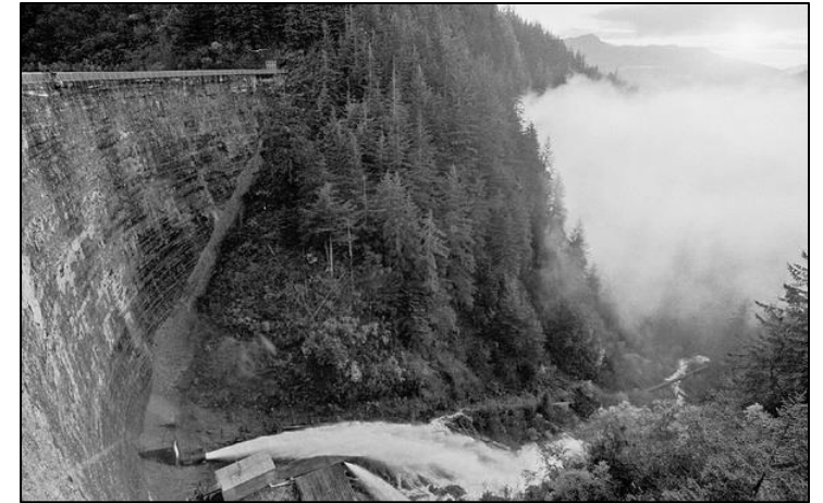
The Salmon Creek Dam provides power to Juneau, Alaska, one of several remote microgrids serving the state.
