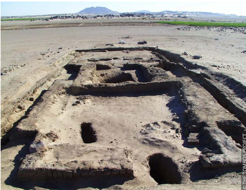
The foundations of Siamun's pyramid; one of ten in the elite Tombos cemetery.
