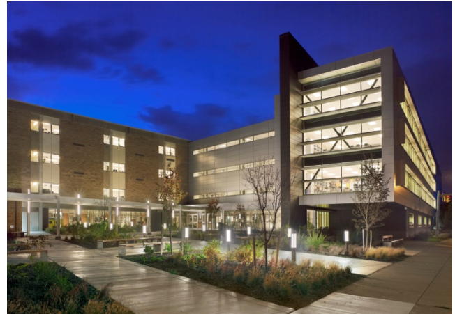
Buffalo Public Schools PS305 exterior addition and renovation completed in Phase IV.
