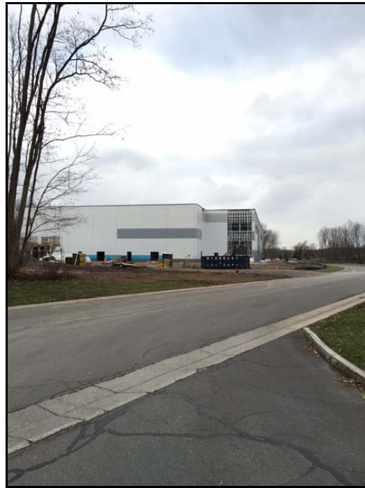
Construction of the future Soraa Facility near the subject
