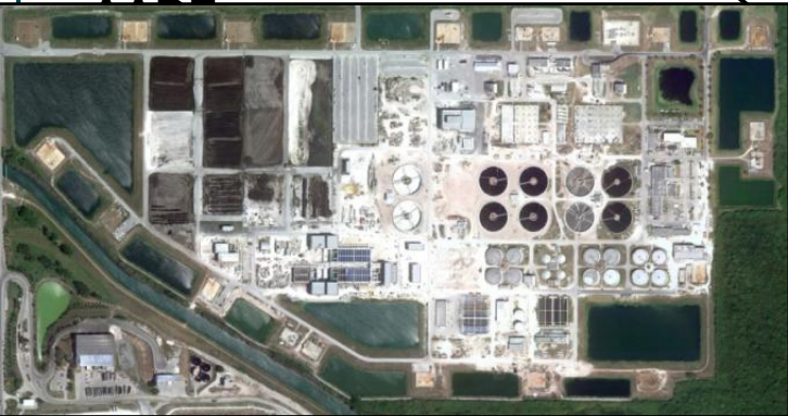
SDWWTP – 112.5 mgd AADF
