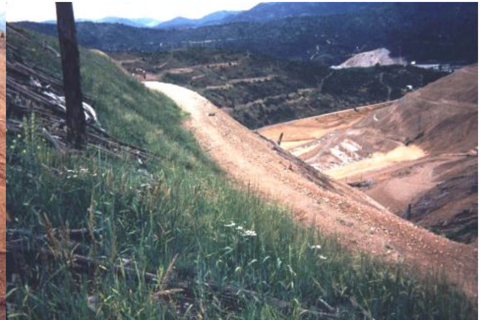
Bunker Hill, ID mine 2 years after reclamation with a blend of biosolids, wood ash, and logging debris.
