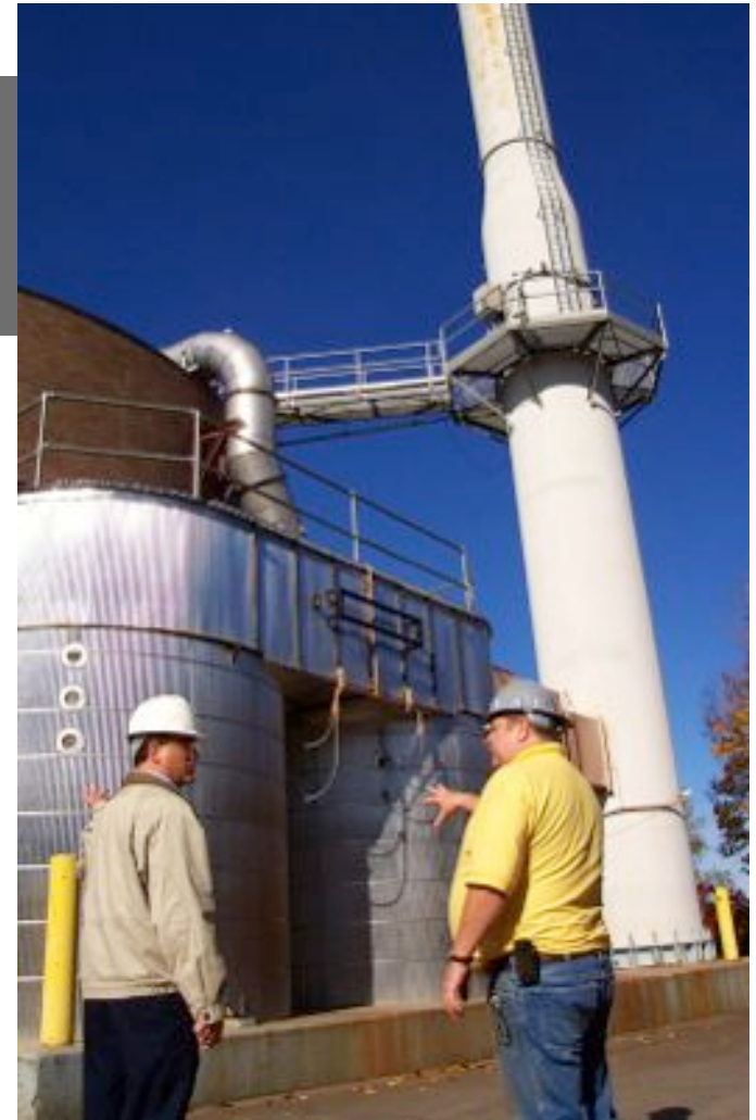
New Haven incinerator, operated by Synagro, with energy recovery.
