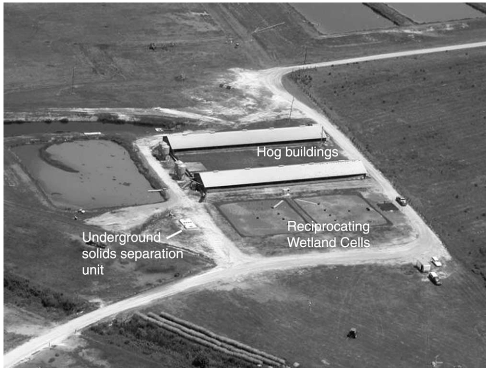
Fig. 2. Aerial view of the reciprocating wetlands system.
