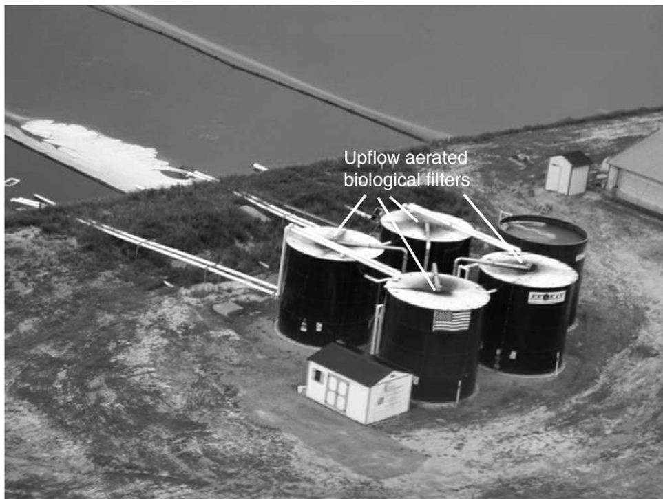
Fig. 3. Aerial view of the upflow aerated biological filter system.
