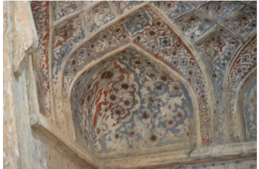
8 Squinches acting as structural as well as aesthetical elements
