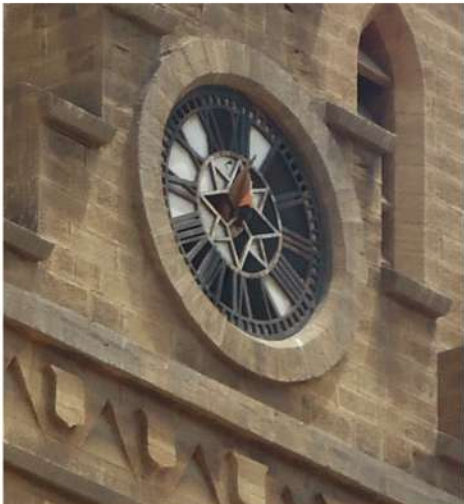
A close up of the neglected rusted condition of the clock. The hands of the clock are missing while the dial is broken.
