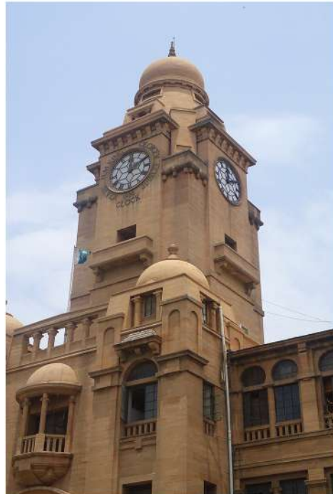
A view of the KMC clock tower from M.A. Jinnah Road.
