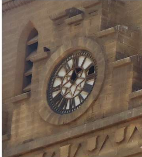
A close up of the neglected rusted condition of the clock. The hands of the clock are missing while the dial is broken.
