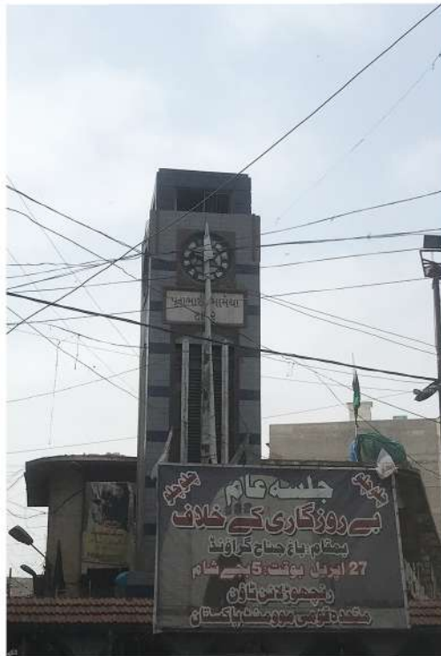
The clock is in a neglected state, blocked by banners and poles resting on it.
