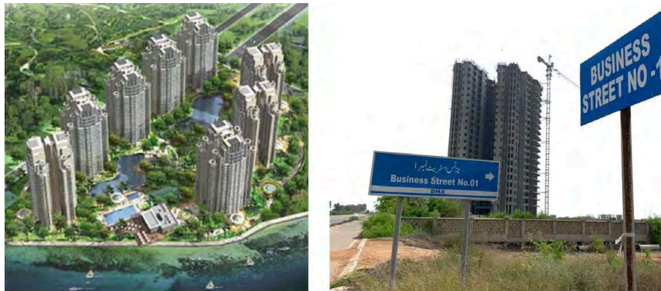
Creek Marina plans, alongside an image of what it looks like currently from site visit. Source: http://www.creekmarina.com/theme/about/
