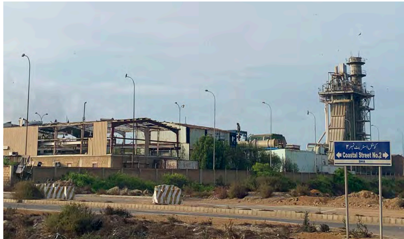
Abandoned DHA Cogen Desalination Plant, DHA Phase VIII
