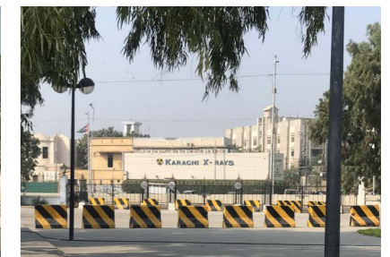
Barriers around the entrances - Javeria Taufiq 2019
