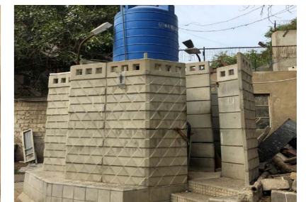
Toilet Facilities - Fizzah Riaz 2019
