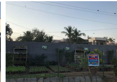
Concrete walls toward neelum colony - Javeria Taufiq 2019
