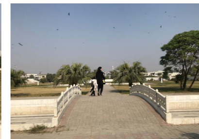
Bridges with dry water bodies - Javeria Taufiq 2019
