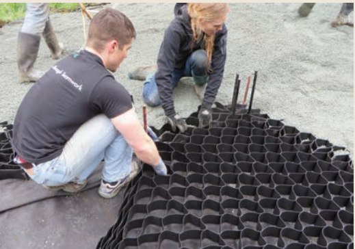
The Lighthoof system in place (above) and being laid out in a paddock (below).
