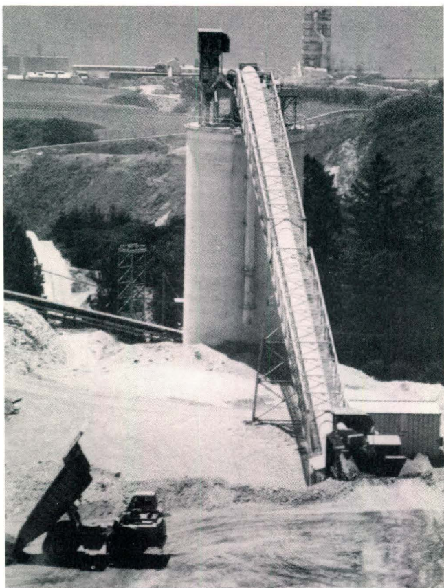
◀ Photo 5. Conveyor and silo at the Bonny Doon shale quarry. The conveyor from the Bonny Doon limestone quarry is to the left of the silo. Main plant is in the distance.
