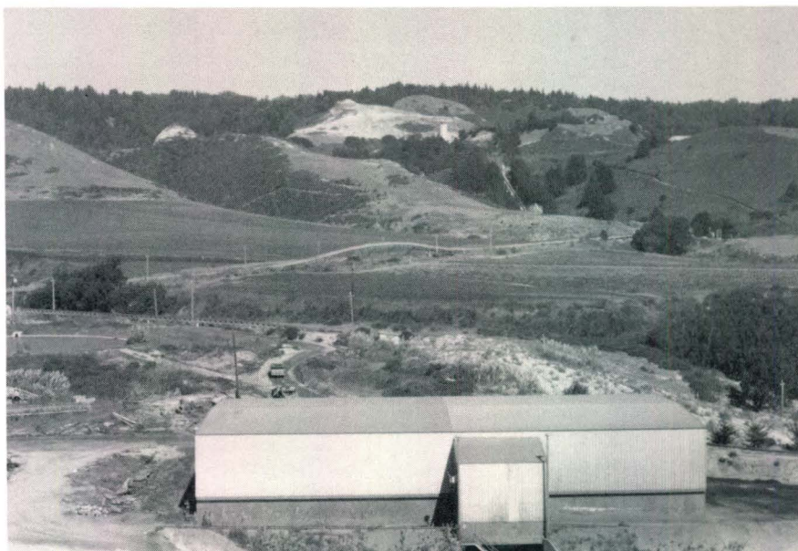
Photo 7. Warehouse building where the limestone and shale are stored. The Bonny Doon shale quarry, silo, and conveyor belt system are visible beyond the warehouse. When needed, the limestone and shale are transported by conveyor from the warehouse and processed.
