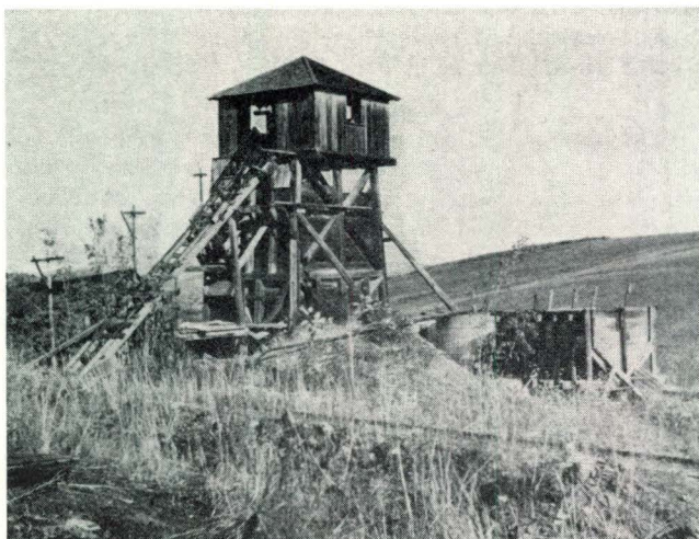
Head frame at Cleveland-Pacific mine (formerly Escondido), circa 1897. Photo from Division of Mines and Geology Archives.
