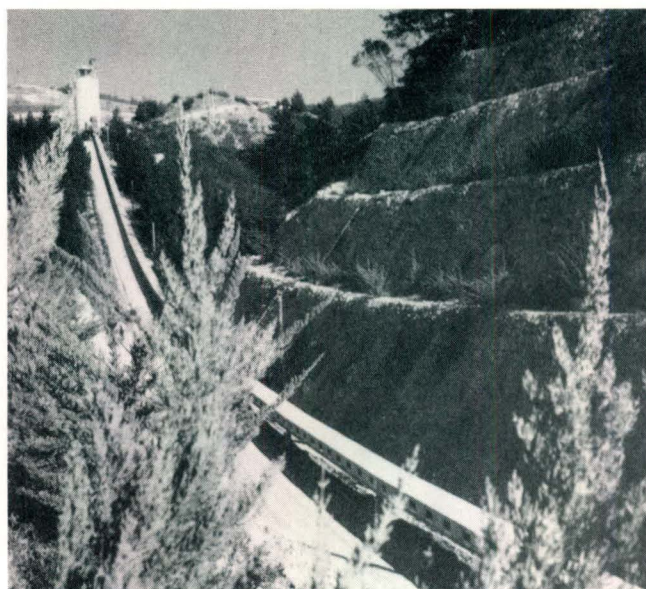
▲ Photo 6. The conveyor belt system which transports limestone and shale from the quarries is housed in concrete to minimize dust emissions. Storage silo at the Bonny Doon limestone quarry is on the hill to the left.
