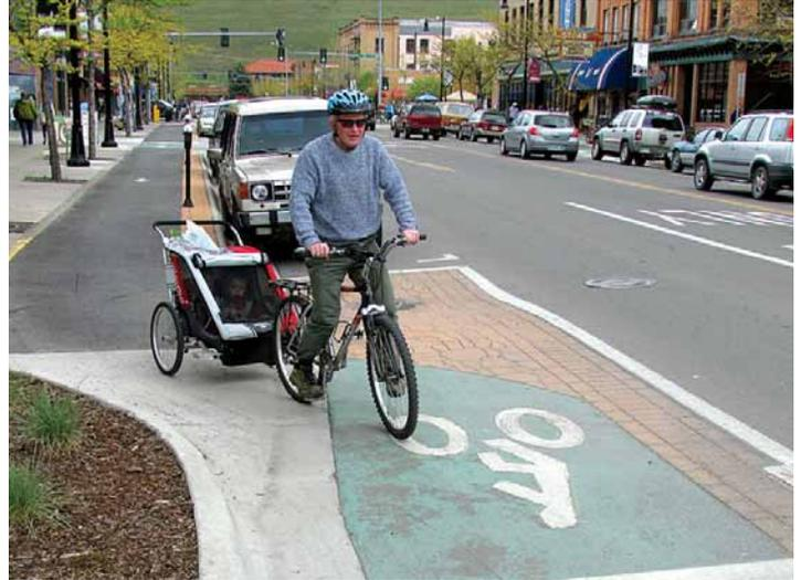
Grade-separated, protected bike lanes (like this raised cycle track in Missoula, Montana) provide separate, defined spaces for riders and drivers.
