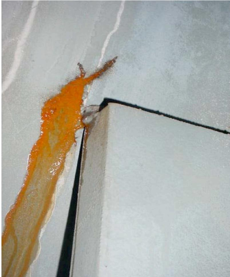
As a result of questions during the ACRS discussion period relating to BWR thick containment designs like the through wall cracks at Hatch 1 and 2, Fairewinds researched additional failures and found that the Fitzpatrick nuclear power plant developed a large though-wall leak that was not due to corrosion. Once again, here is a unique violation of the BWR containment system that is directly applicable to the Westinghouse design of the AP1000.
