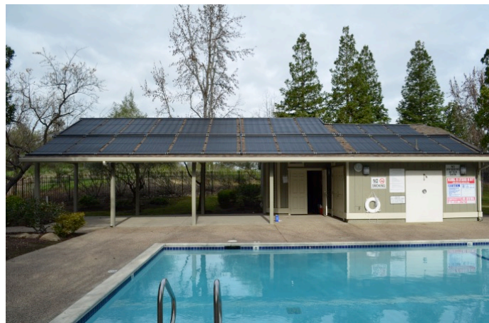
Figure 11. Typical uninsulated polymer pool panel (left) and installed commercial system (right).
