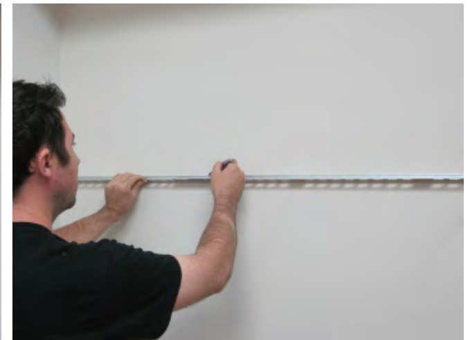
STEP 3: Draw horizontal reference lines on wall, or use a laser to level the row of tiles to be installed. Repeat this step for each new row.
