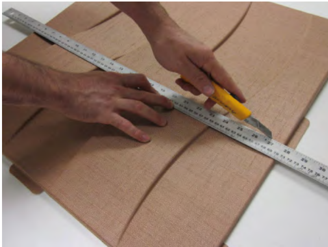
STEP 13: Cut the tile to the required size using a utility knife.
