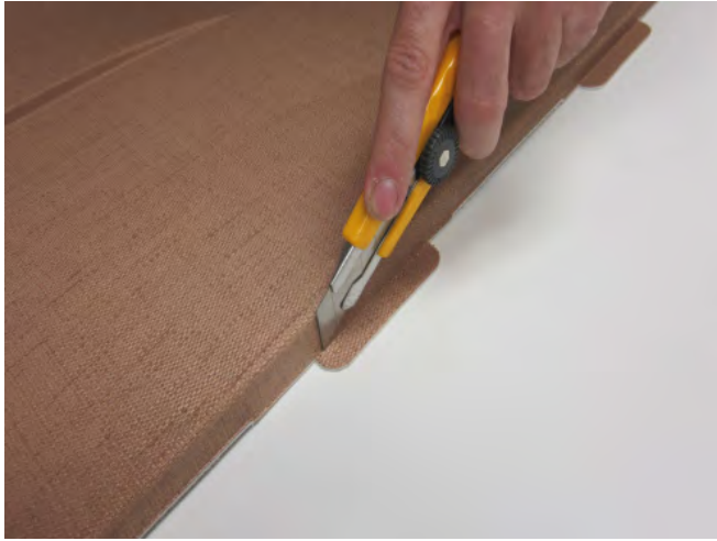
STEP 4: Cut the tabs off the identified files on your plan that will go along the trims, by using a utility knife or scissors.
