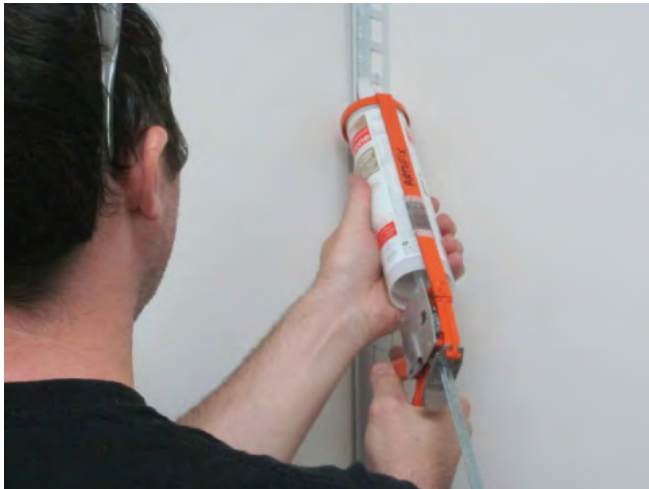
STEP 7: For the tiles that will fit onto trim ARTOTRIM-L1, use a transparent silicone caulking to fasten them into the trim.
