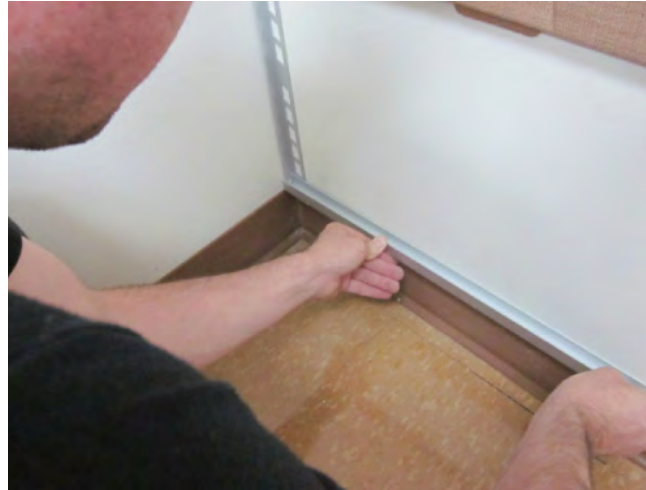
STEP 11: Firmly press the ARTOTRIM-C1 against the wall and add screws to fasten the trim to the wall.
