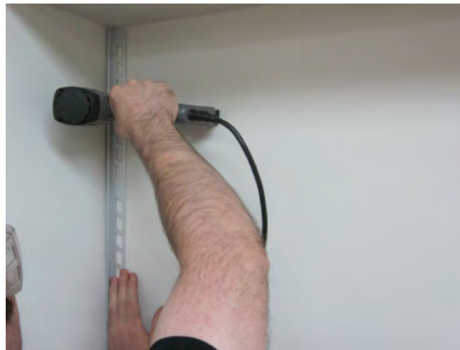
STEP 2: If desired, fasten the trim to the wall by using screws or 12 mm (½") staples.
