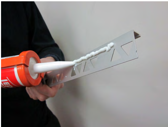
STEP 1: Add adhesive caulking on the rear of the ARTOTRIM-L1 trim and affix to the wall.
