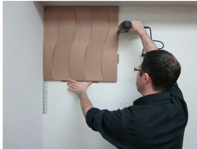
STEP 8: Put the first tile on the ARTOTRIM-L1, staple all the visible tabs on the file. Make sure the tiles are aligned.
