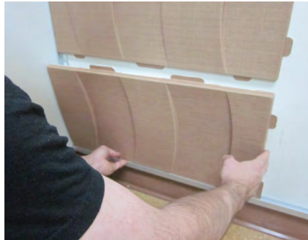
STEP 14: Insert the file bottom in the ARTOTRIM-C1 and strips in the upper files.
