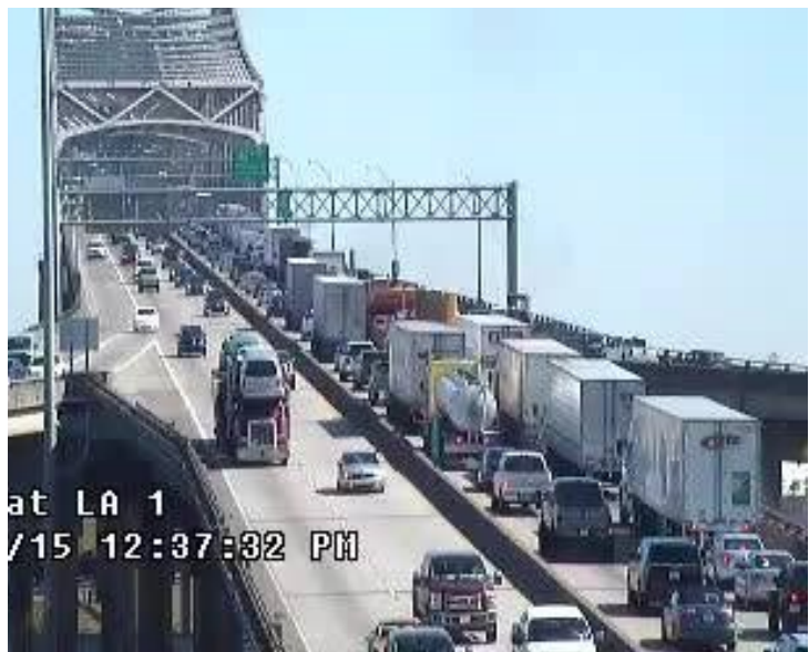
DOTD traffic cameras show heavy delay along I-10 in West Baton Rouge Parish at the Mississippi River bridge. Alleviating this congestion is a top priority for state, local, and regional leaders.
