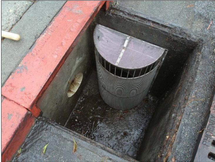
Figure 2.2. Example small full-capture device used as a monitoring site.
