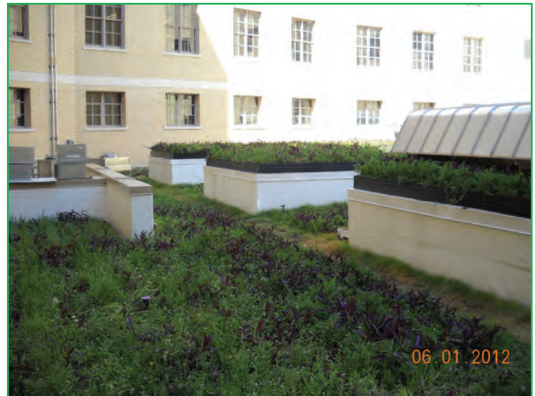
LiveRoof Texas Project Installation San Antonio, TX 6.01.12
