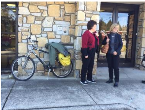
Cracked sidewalks in need of repair
