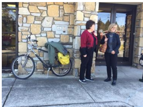
Cracked sidewalks in need of repair
