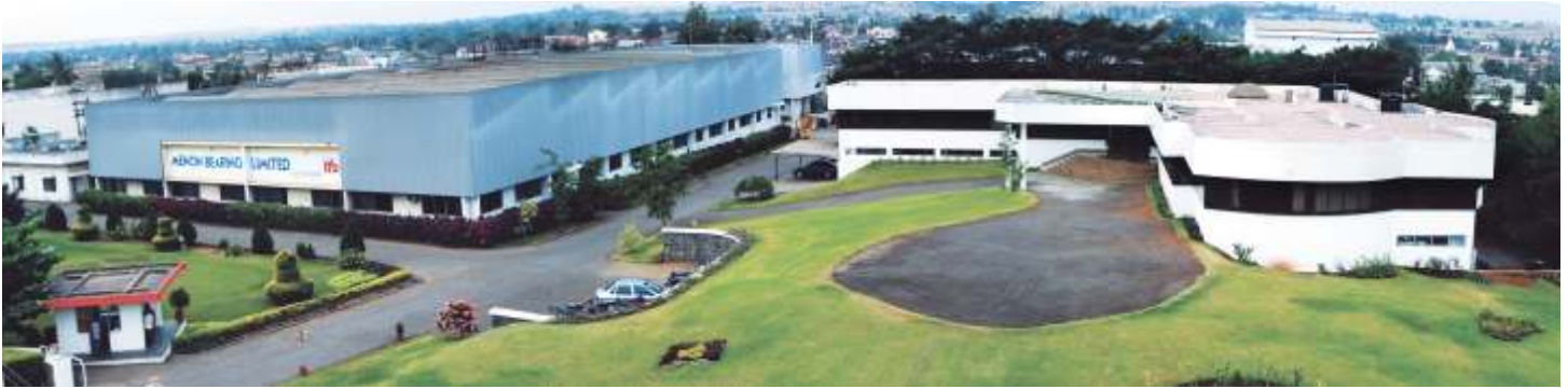
Bearings Manufacturing facility at MIDC, Gokul Shirgaon, Kolhapur, INDIA.
