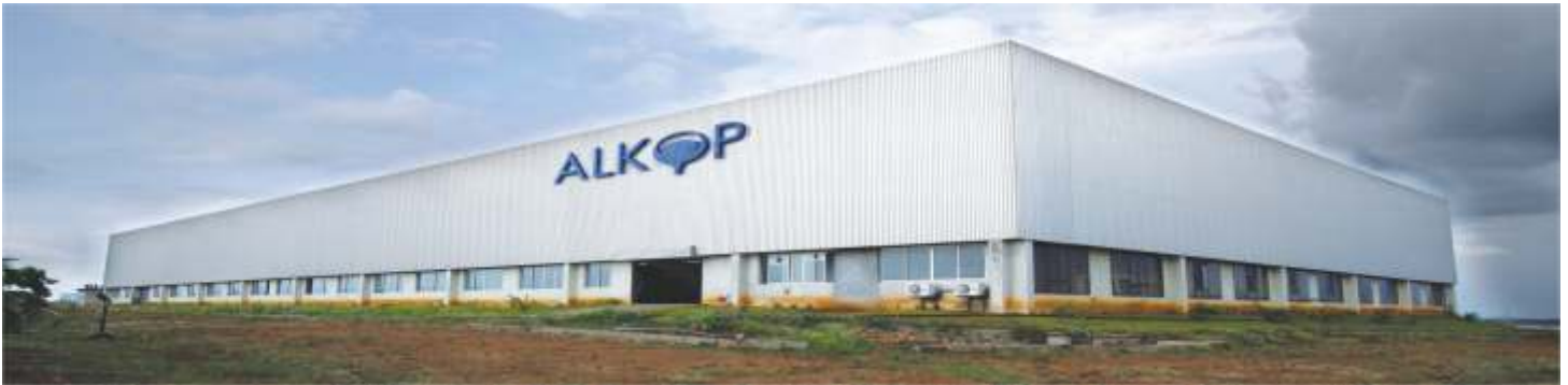
Aluminium Division Manufacturing facility at MIDC, Kagal, Kolhapur, INDIA.
