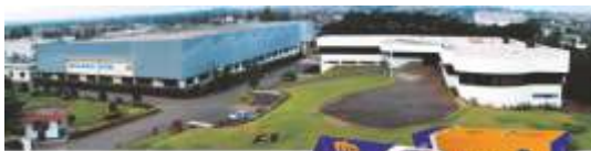
Menon Bearings plant at Kolhapur,
