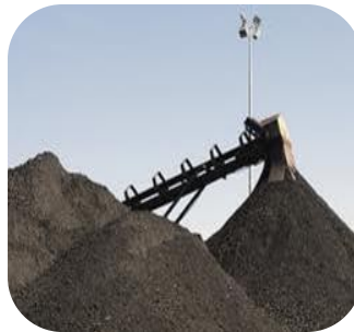
POWER PLANT COAL PILE
