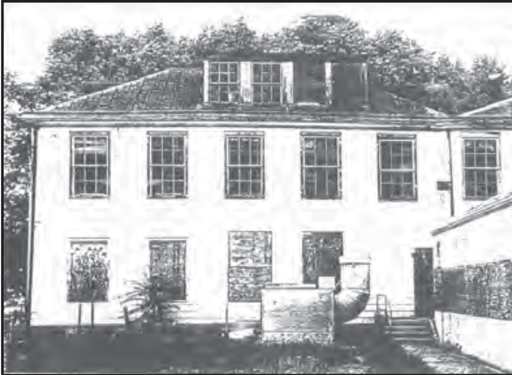
Plate 3.15. View of the southern façade of Rosey Hill Mansion. 1975. (Source: New Jersey Department of Transportation 1975).
