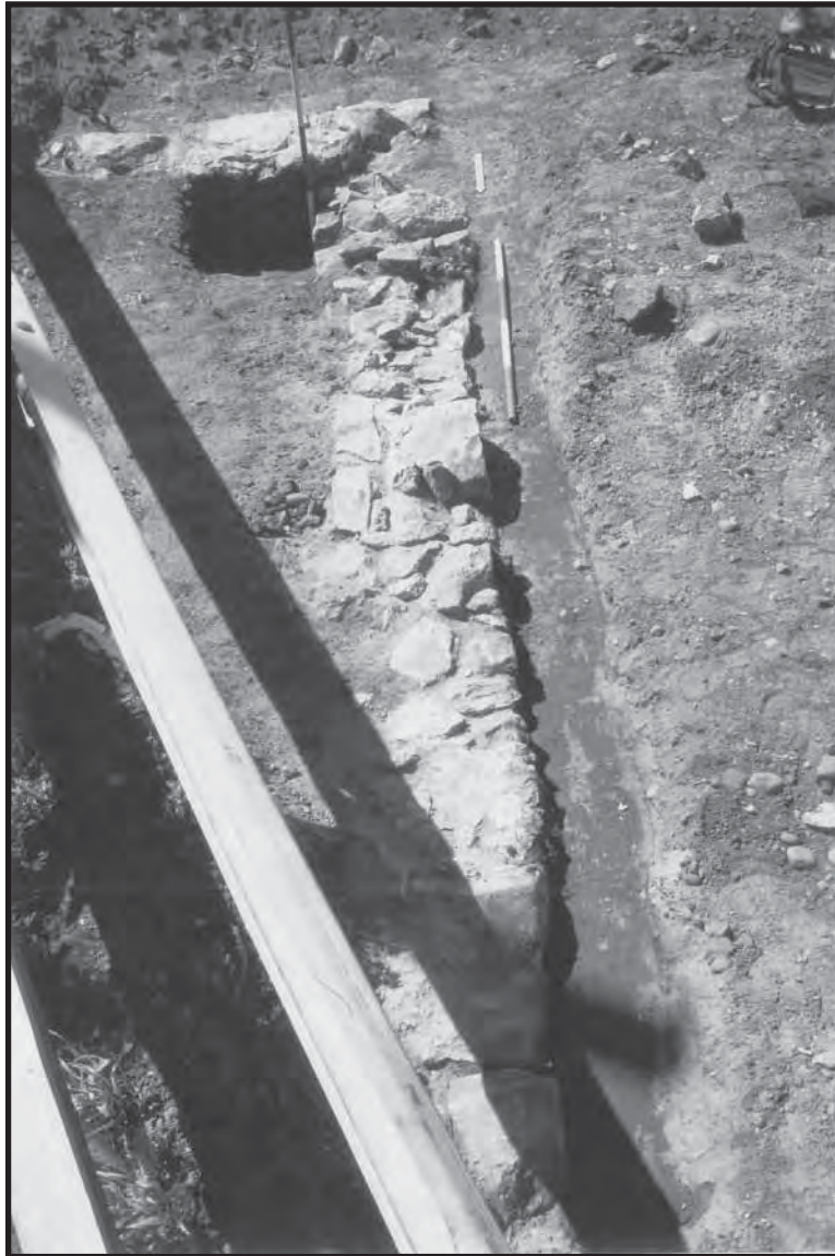
Plate 4.129. Lambert/Douglas Plantation and Rosey Hill Mansion Site: view looking south showing New Jersey Steel and Iron Company chain drying shop foundation; scales in feet and inches (Photographer: George D. Cress, July 1999) [HRI Neg. #99011/9:20].
