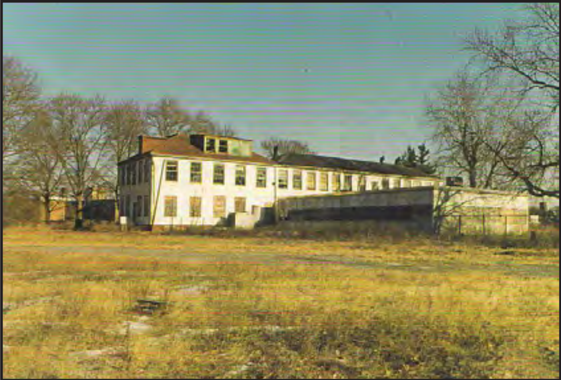
Plate 3.18. Historic photograph of Rosey Hill Mansion just prior to demolition, looking north and east. Circa 1980. (Source: New Jersey Department of Transportation).
