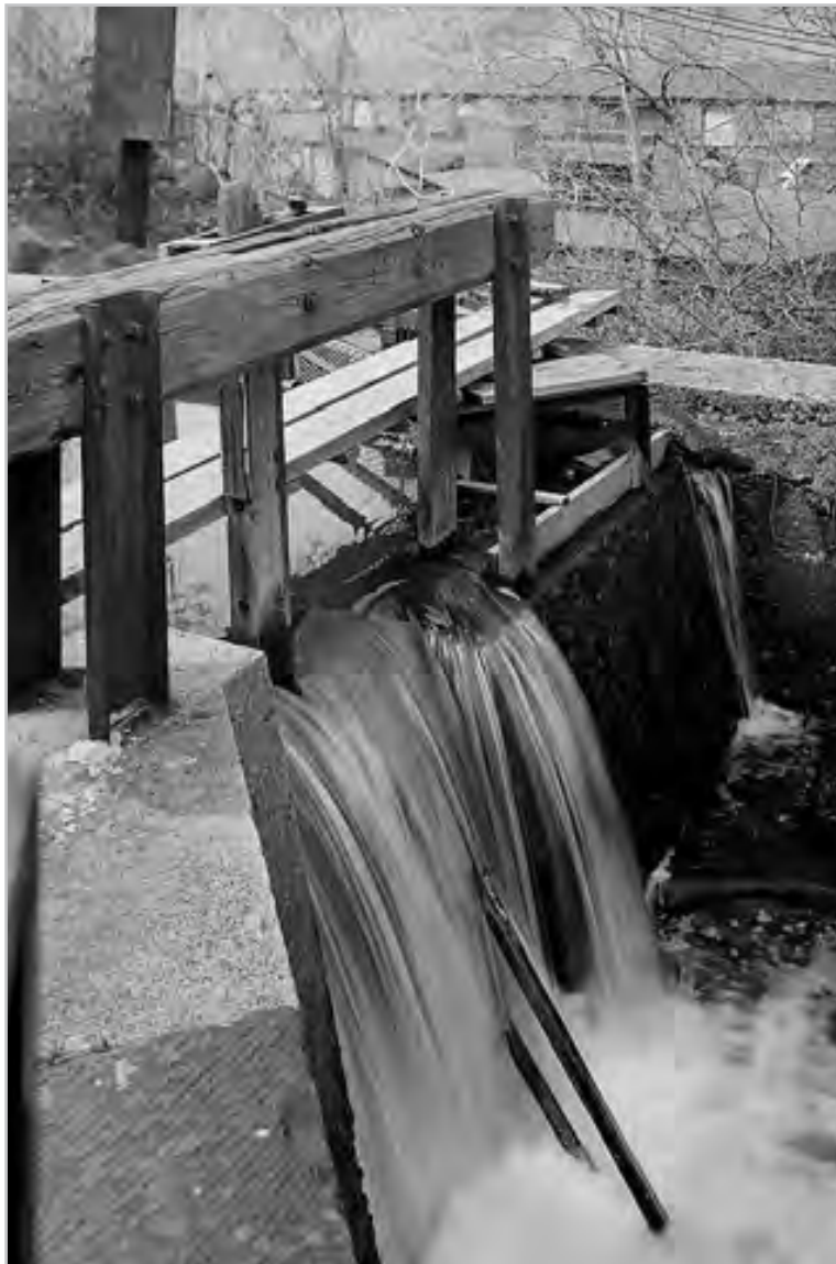
Plate 5.6. The spillway gate at the north end of the Middle Raceway, located between the Essex Mill and the Gun Mill, view looking north northwest, 1974. In earlier times, there was a gatehouse located to the east of this gate. This was an important point for regulating the flow and height of water in the Middle and Lower Raceways. The S.U.M. attempted to keep a sounding (depth) of water of 3 feet in the raceways to meet its contractual obligations to supply water for power. Source: Historic American Engineering Record, HAER NJ-2, 1974.
