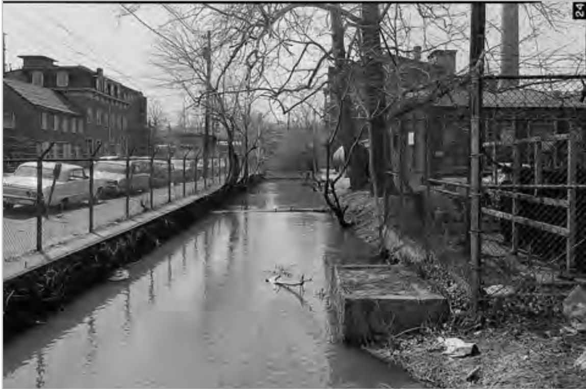
Plate 5.5. The Lower Raceway, looking west, 1974. The headrace for the Todd Mill begins at the concrete gate structure in the foreground at right. Source: Historic American Engineering Record, HAER NJ-2, 1974.
