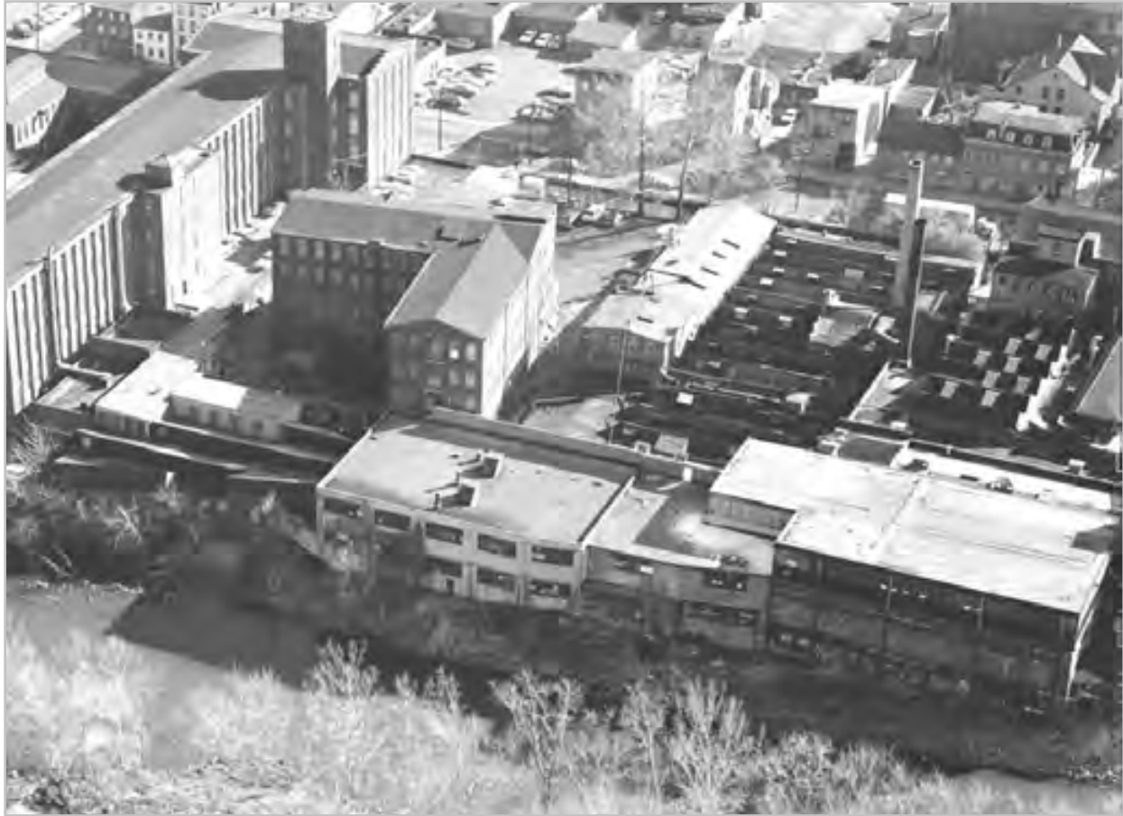
Plate 3.52. Aerial view of the Allied Textile Printing site looking south southeast showing the rear yards of the Todd and Rafferty Machine Company works and the Passaic and Waverly mills, 1973. Source: Historic American Engineering Record, HAER NJ-1-26, 1973.
