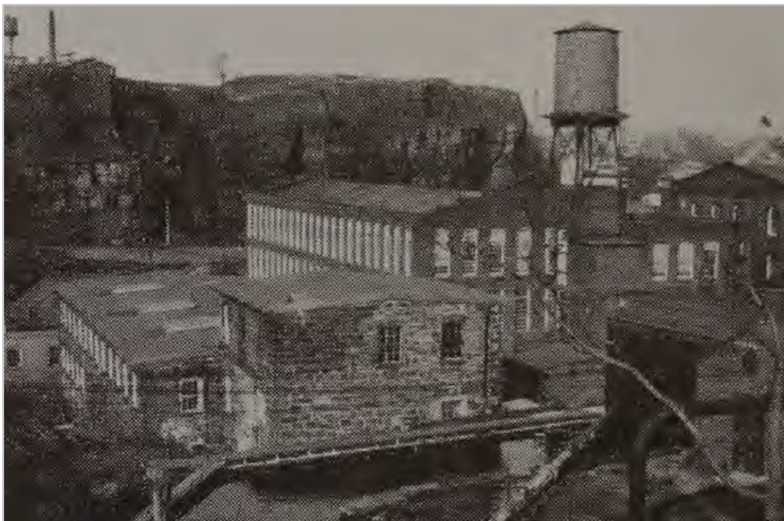
Plate 5.2. View of the Middle Raceway looking north toward the Gun Mill, circa 1927. Note the gatehouse (right). The S.U.M. steam pipe is also visible. It was installed circa 1916 to supply steam from the S.U.M. steam plant (at what is now Overlook Park) to the Mallory/Waverly mill complex. Source: Heusser 1927.
