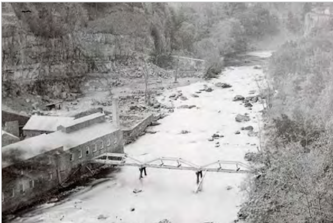
Plate 5.10. View looking south southwest and upstream showing the “Broomstick Bridge,” circa 1865. The broomstick bridge carried the Passaic Water Company’s water supply line. Source: Paterson Historic Preservation Commission.
