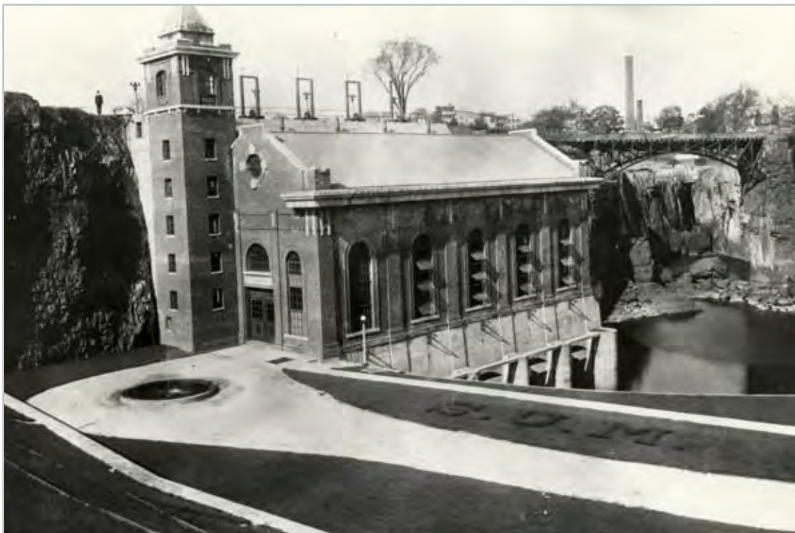
Plate 5.14. The S.U.M. Great Falls Power Plant, looking west, circa 1915. The hydroelectric plant opened in 1914. Electrification allowed the S.U.M. to convert the mills from waterpower to electricity, with a substantial savings in water, since the power plant could produce as much power with half the water. It was a major factor in the abandonment of the direct-drive mill water and steam-power systems at the ATP site. Source: Paterson Museum Collection 2009.
