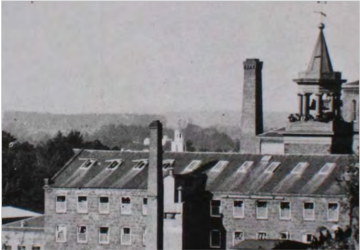
Plate 3.9. Detail of photograph of circa 1860 showing the Gun Mill. The mill's rifle-shaped weathervane is visible surmounting its cupola. The large chimney was attached to the mill's boiler house. The skylights visible in the mill's roof were probably those installed in 1846 to facilitate the use of the fifth floor of the mill for silk manufacture (Trumbull 1882:173). Source: New Jersey Historical Society, Manuscript Group 1361.
