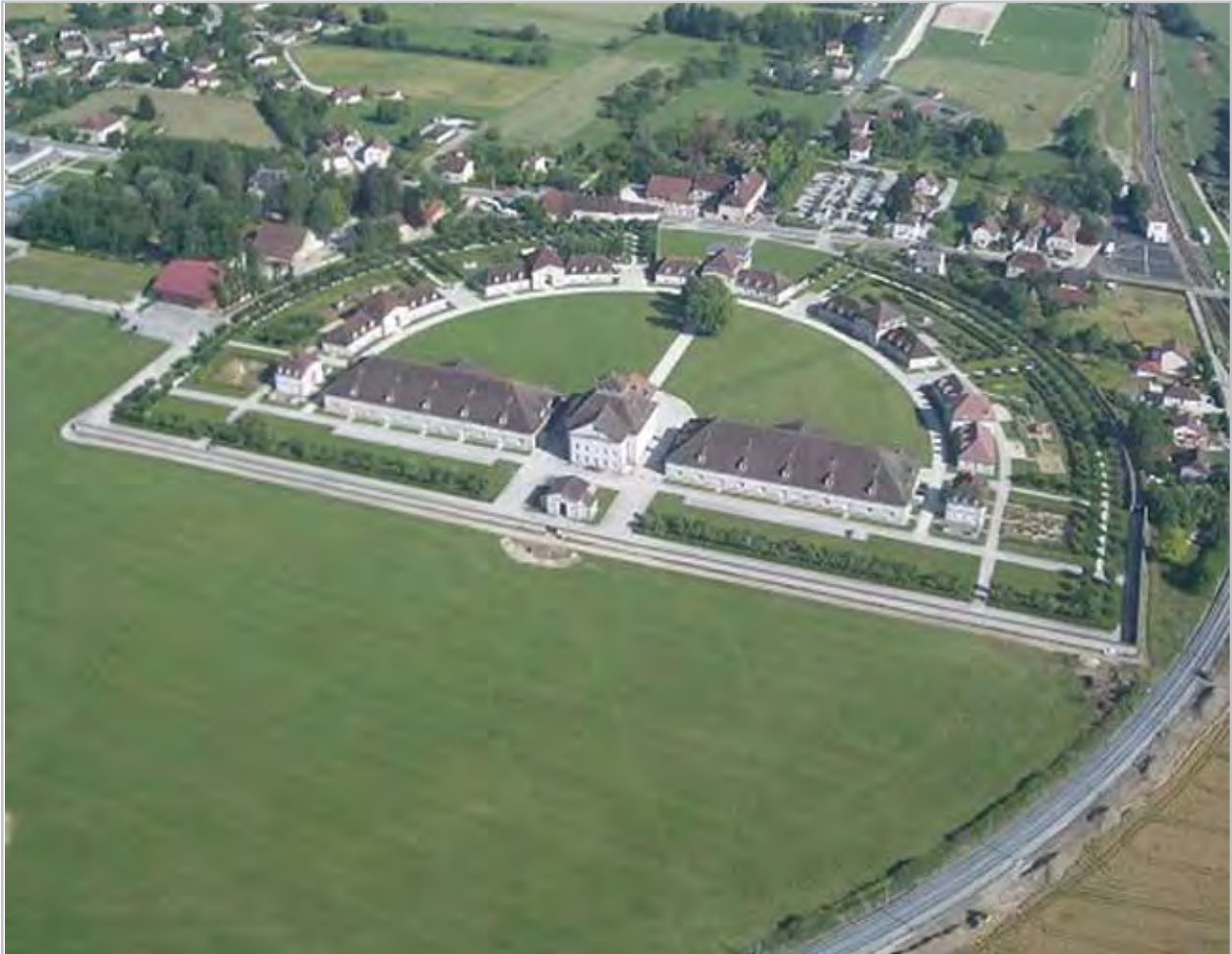
Plate 2.6. Photograph of the Saline Royale at Arc-et-Senans. Most of the buildings of the planned community which was to surround the royal salt works were never constructed. Several of those that were built have not survived to the present day.
