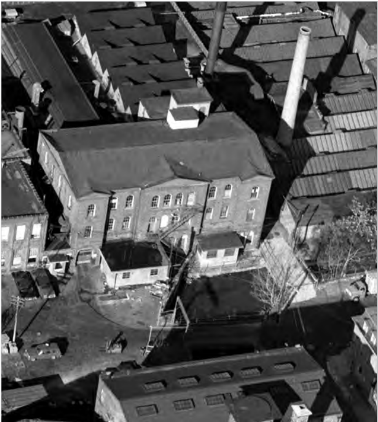
Plate 3.50. Aerial view of the Waverly Mill looking north northeast, 1973. Source: Historic American Engineering Record, HAER NJ-1-9, 1973.
