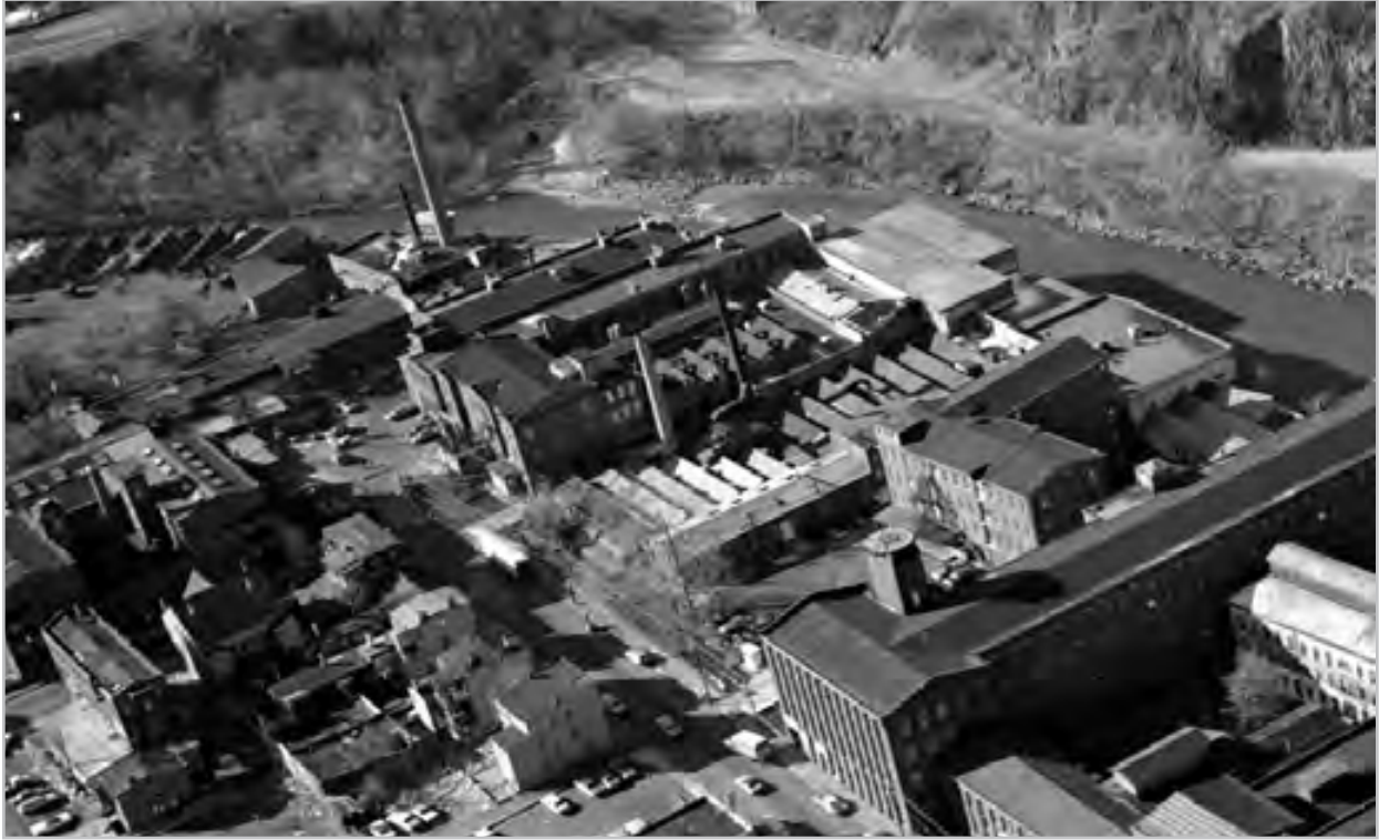
Plate 3.46. Aerial view of the Allied Textile Printing site looking west northwest, 1973. Source: Historic American Engineering Record, HAER NJ-1-6, 1973.
