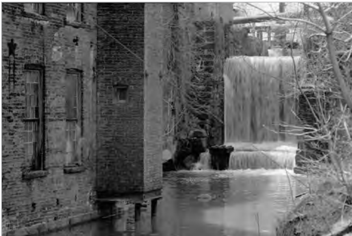
Plate 5.7. View of the spillway between the Middle Raceway (far) and the Lower Raceway (near), looking west southwest, 1974. The top of the first fall appears to be the location of an earlier S.U.M gatehouse; the gate beyond was added later, probably after 1930. Source: Historic American Engineering Record, HAER NJ-2, 1974.
