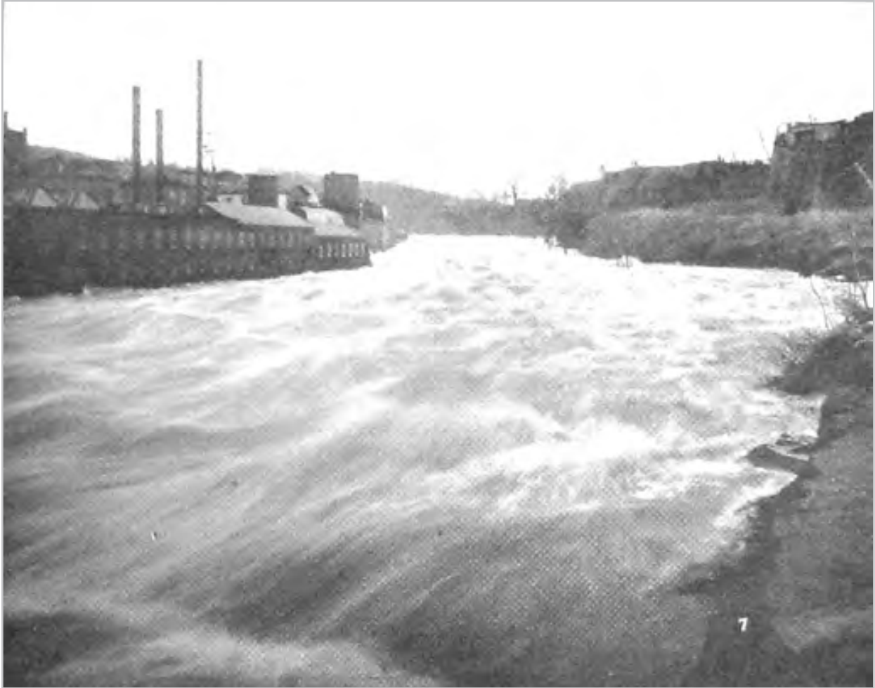
Plate 3.23. View looking southwest and upstream showing the Passaic River and the Knipscher & Maass Silk Dyeing Company works during the flood of March 3, 1903. Source: Paterson Evening News 1915.
