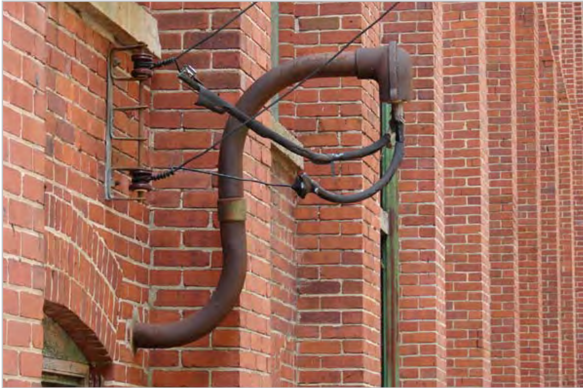
Plate 5.15. Electric drop on a silk throwing mill, 2007 [Klotz Throwing Mill, near Cumberland, Maryland]. The electric drops at the ATP site are now in the rubble, but electrification allowed for electric lighting and the powering of machines by individual motors. Source: Patrick J. Harshbarger 2009.
