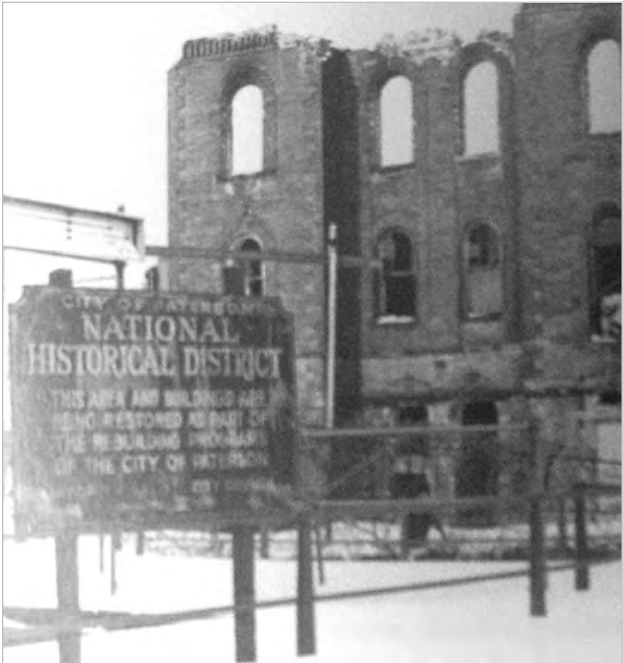
Plate 3.58. View looking north showing the Waverly Mill following the fire of 1983. Source: Avignone 1999.
