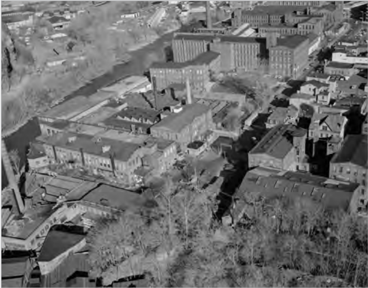
Plate 3.43. Aerial view of the Allied Textile Printing site from above Mount Morris looking north northeast and downstream, 1973. Source: Historic American Engineering Record, HAER NJ-1-8, 1973.
