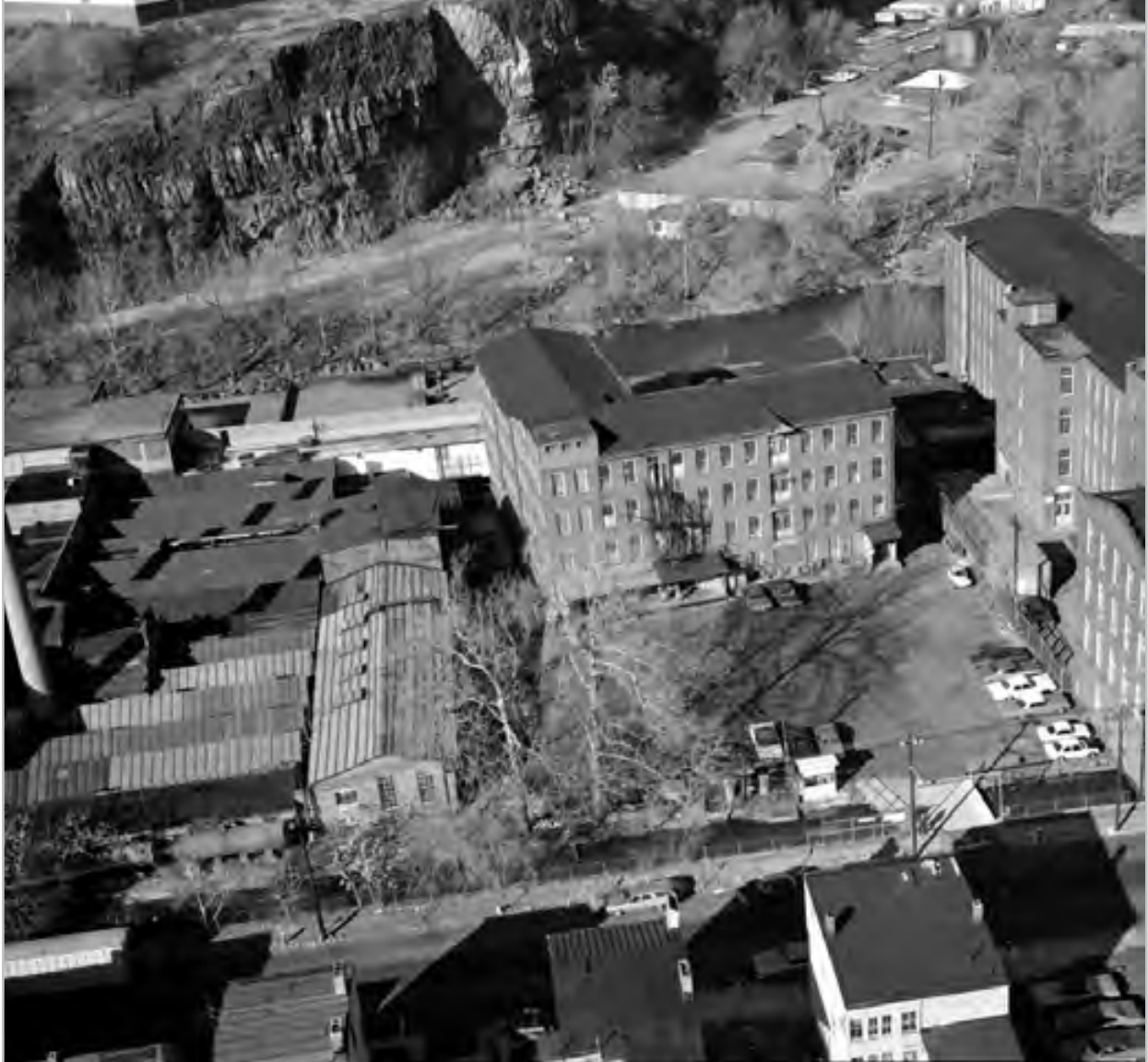
Plate 3.53. Aerial view of the Todd and Rafferty Machine Company works looking north, 1974. Source: Historic American Engineering Record, HAER NJ-5-1, 1974.
