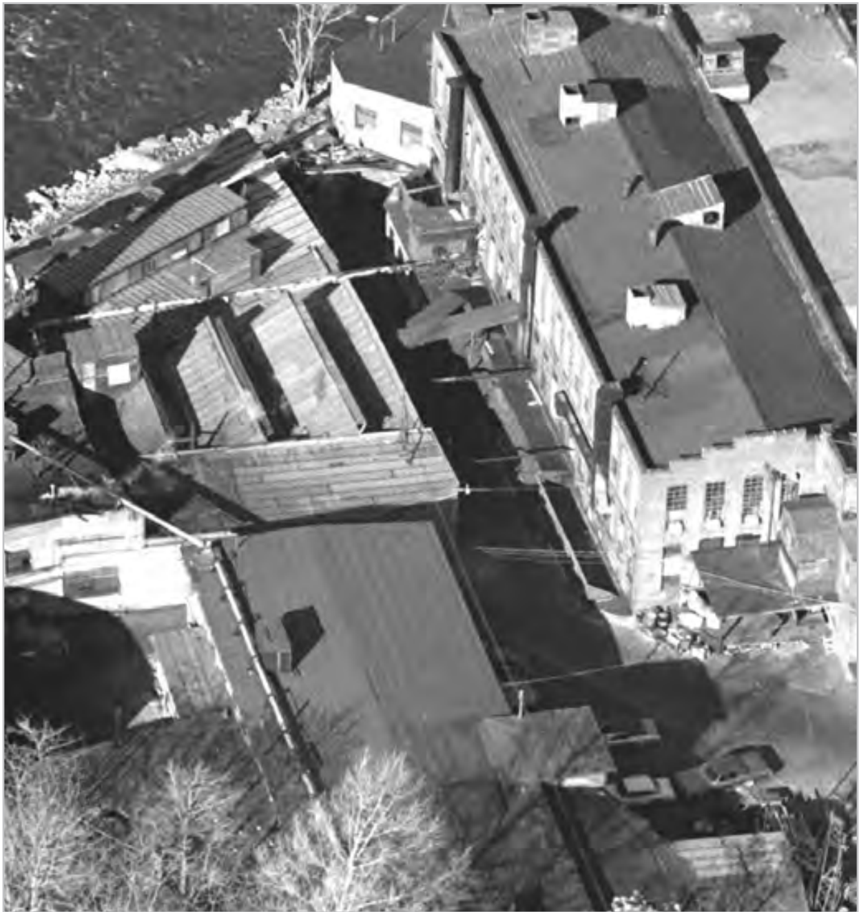
Plate 3.49. Aerial view showing the Gun Mill, 1973 [bottom and left] and the Mallory Mill [top and right], looking north, 1973. Source: Historic American Engineering Record, HAER NJ-1-9, 1973.
