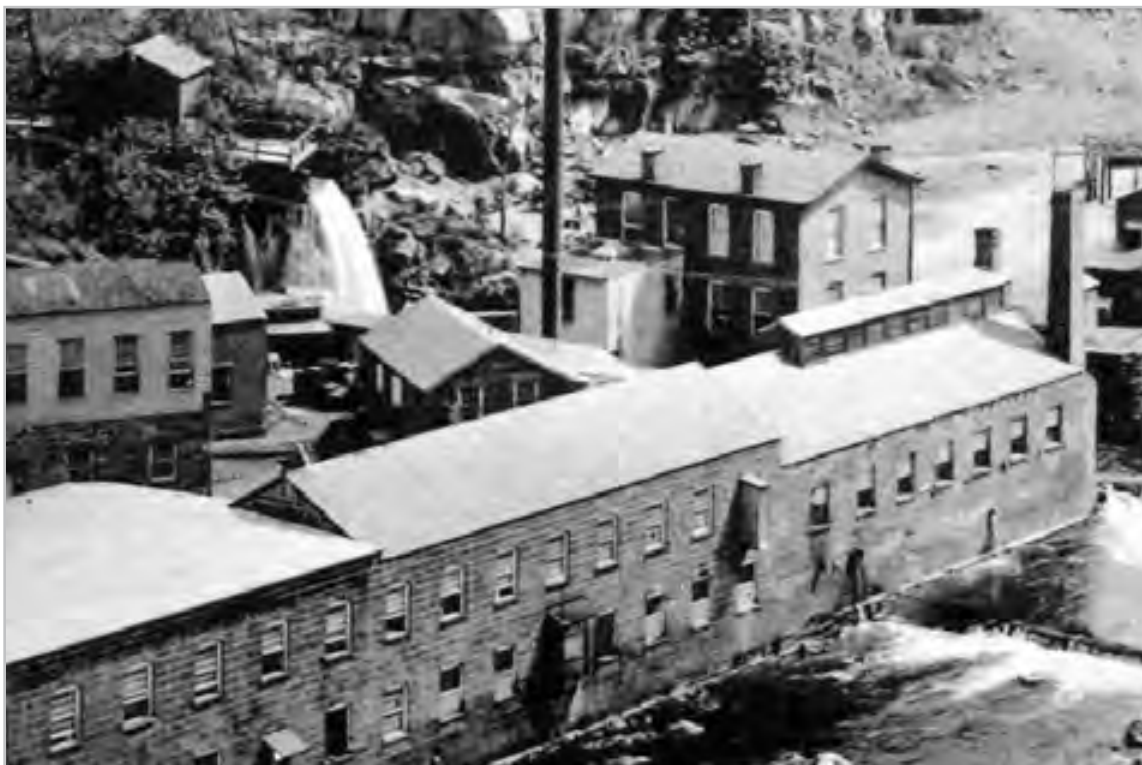
Plate 5.4. Undated early 20th-century view looking south showing detail of the North Gates Waste Way. This flume and gatehouse allowed the S.U.M. to release excess water from the Middle Raceway to the Passaic River. It was one of two control points at the north end of the Middle Raceway; the other fed the Lower Raceway (see Plate 3.3). Source: Paterson Historic Preservation Commission.
