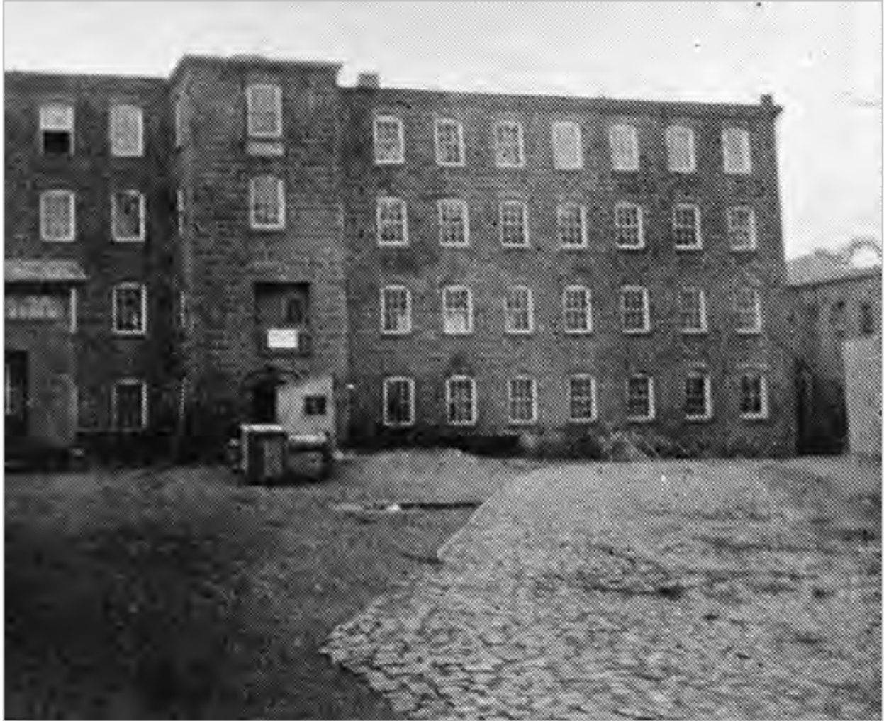
Plate 3.28. View of the Gun Mill, looking west, circa 1910. This image shows the cobble-paved yard in front of the mill and loss of the upper story of the building. Source: Heusser 1927:178.
