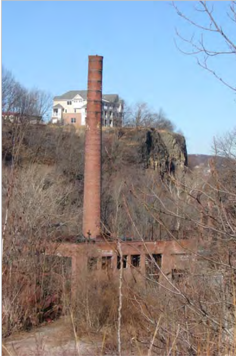
Plate 5.11. Standard Boiler House. Source: Patrick Harshbarger, 2009.
