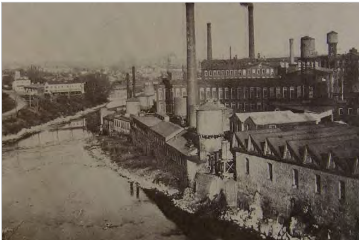
Plate 5.1. The ATP site, looking northeast and downstream from the Great Falls, circa 1927, by which time the site was largely devoted to textile dyeing and printing. Note the numerous roof-top water tanks. The tanks in the top right corner were installed circa 1908 to supply fire sprinkler systems in the Mallory and Waverly Mills. The smokestack with the SSD initials marks the location of the “Standard” boiler house. Source: Heusser 1927.
