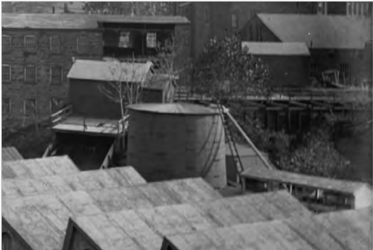
Plate 3.25. Detail of historic photograph of “Paterson, N.J. from Water Works Park” showing the Gun Mill flume and gatehouse structure, circa 1904. Source: Detroit Photographic Company.
