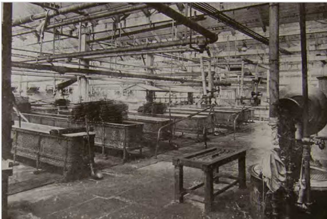
Plate 5.12. Interior view of the Standard Silk Dyeing Company, circa 1927. Note the numerous pipes for delivery of steam and water. Source: Albert H. Heusser, The History of Silk Dyeing Industry in America , 1927.
