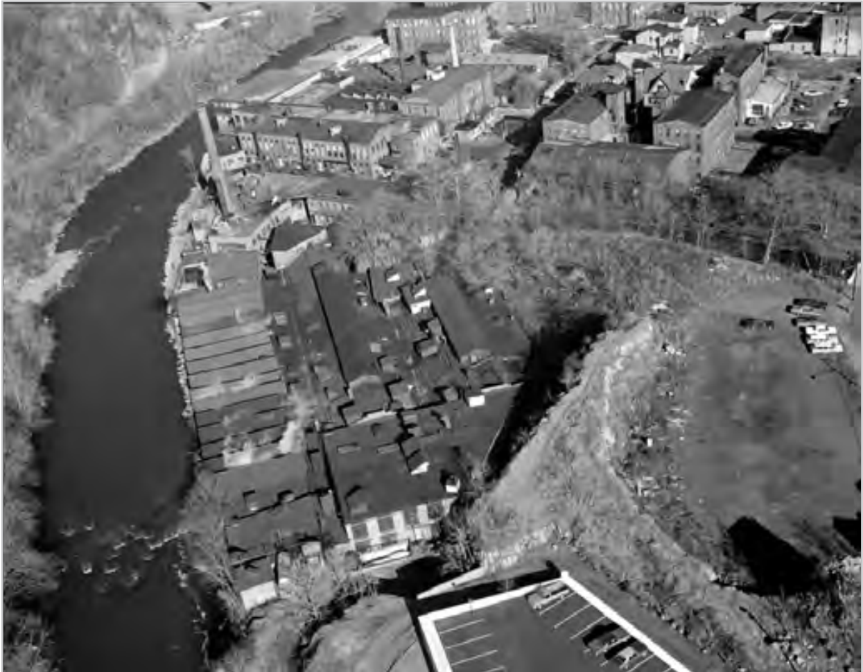
Plate 3.42. Aerial view of the Allied Textile Printing site from above Mount Morris, looking northeast and downstream, 1973. Source: Historic American Engineering Record, HAER NJ-17-1, 1973.
