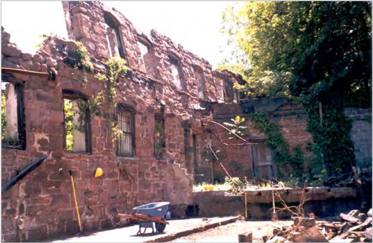
Plate 3.59. View looking northeast showing the Gun Mill prior to stabilization, circa 2000. Source: Paterson Historic Preservation Commission.
