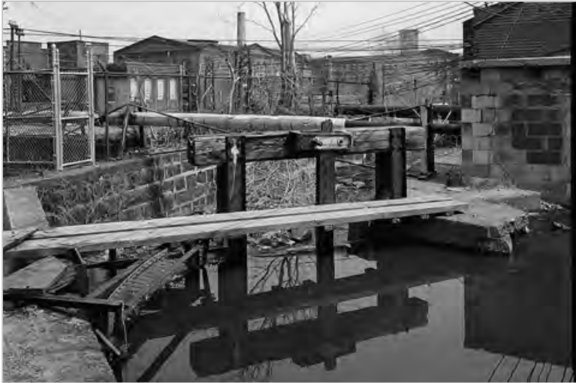
Plate 5.3. The spillway gate at the north end of the Middle Raceway, looking north, 1974. Note the steam lines in the background. These lines connected the Standard boiler house with other mills in the district. Source: Historic American Engineering Record, HAER NJ-2, 1974.
