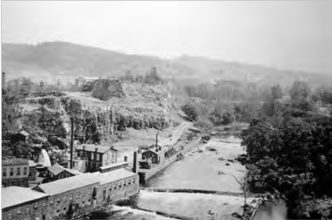
Plate 5.9. View looking south southwest and upstream showing the Knipscher & Maass dye house, North Gates Waste Way, and the quarry, circa 1890. Dams have been placed in the stream to pond water for pumping to supply the Passaic Water Company and the dye house with water. Source: Paterson Historic Preservation Commission.
