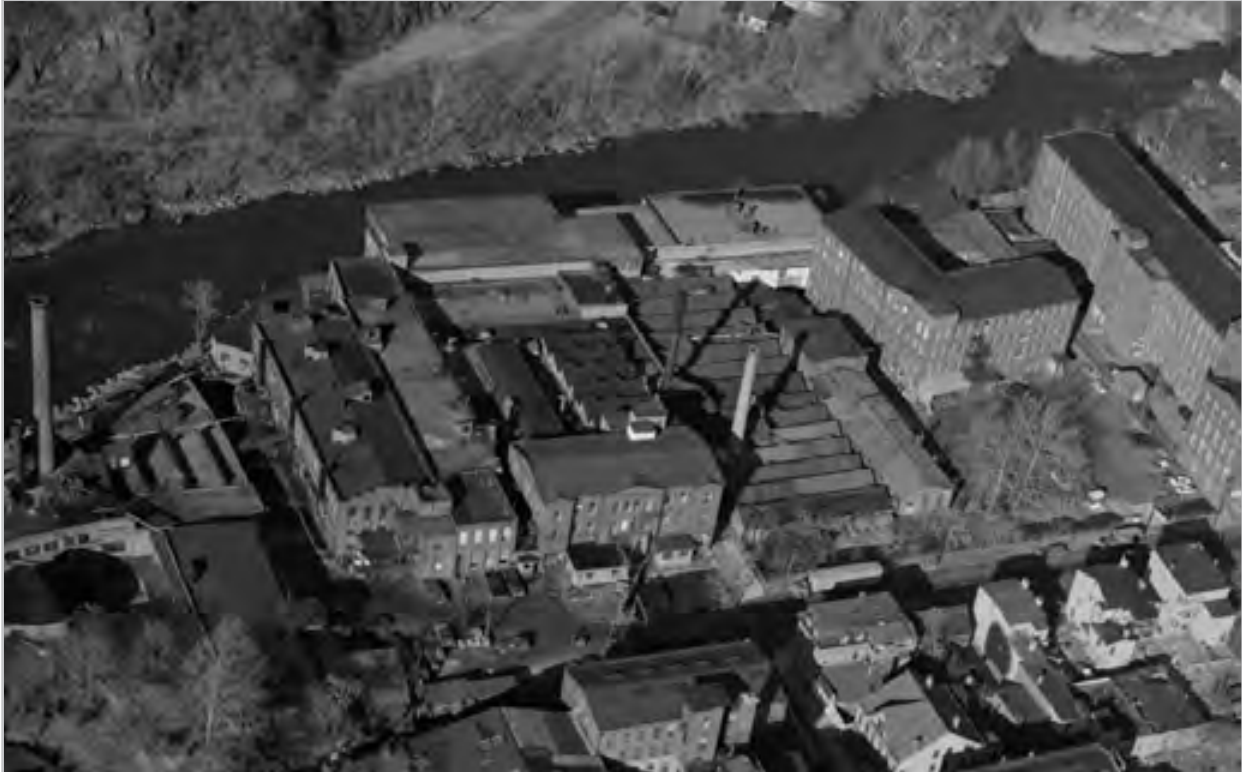
Plate 3.44. Aerial view of the Allied Textile Printing site looking north showing the Mallory, Waverly, Passaic and Todd mills, 1973. Source: Historic American Engineering Record, HAER NJ-1-9, 1973.
