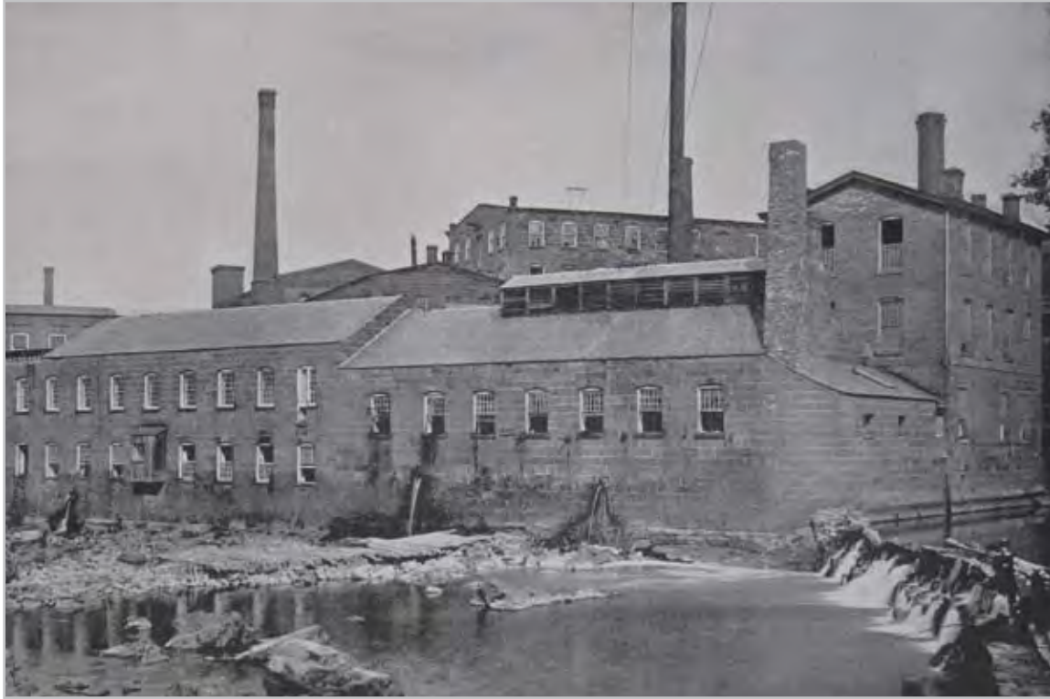
Plate 5.8. Knipscher & Maass silk dye house, view looking east, circa 1890. Note the many pipes and outlets in the river wall and foundation for waste water. The dam (right foreground) was constructed circa 1857 to pond water for pumping by the Passaic Water Company. The three-story structure to the south of the dam is believed to be the pump house, also later used by Knipscher & Maass. Source: Paterson Historic Preservation Commission.
