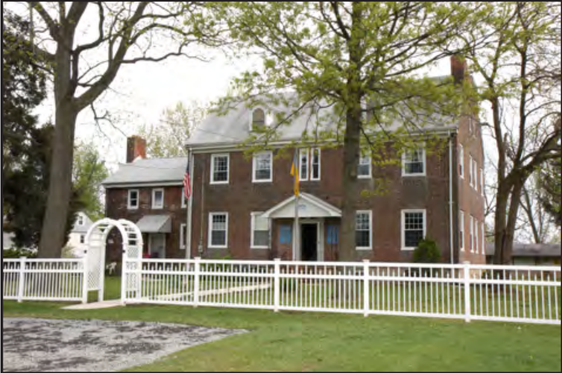
Plate 6.1. Bow Hill, constructed in 1790: view looking south (Photographer: David Byers 2008).
