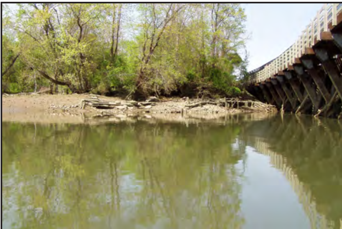
Plate 6.6. The original outlet lock for the Delaware and Raritan Canal, constructed in the early 1830s: view looking north (Photographer: William Liebeknecht 2008).
