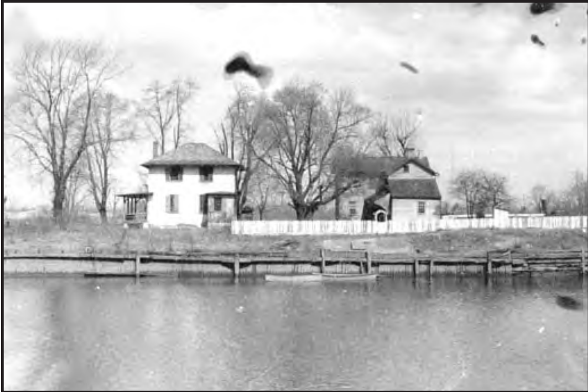
Plate 4.12. Historic photograph of buildings at the Delaware and Raritan Canal Outlet Lock opposite Bordentown. April 1935 (Source: Henry B. Kümmel Collection, New Jersey State Archives).
