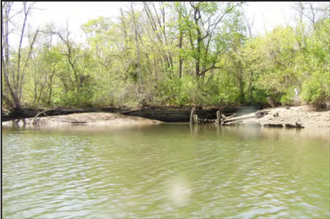
Plate 6.7. The replacement outlet lock for the Delaware and Raritan Canal, constructed in the late 1840s: view looking north (Photographer: William Liebeknecht 2008).
