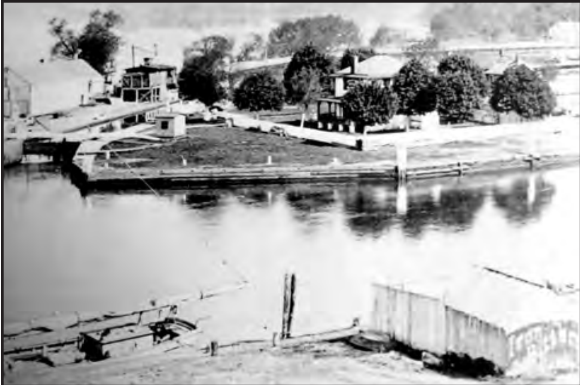
Plate 4.10. Historic photograph of the Delaware and Raritan Canal Outlet Lock from Bordentown. Circa 1886 (Source: McKelvey 1975:10).
