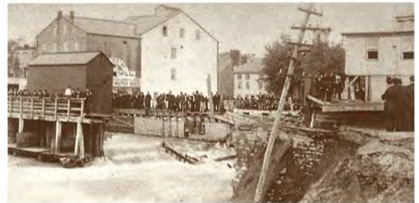
Onlookers view the damage from a September freshet in 1882, which blew out the power canal aqueduct over the Assunpink Creek. [Trenton Public Library]
