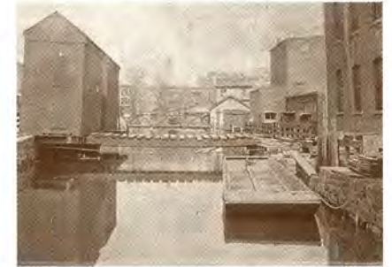
A pair of gatehouses on the aqueduct (at left) controlled the flow of water along the power canal, releasing surplus into the Assunpink Creek below when the water level rose too high. [Trenton Public Library]
