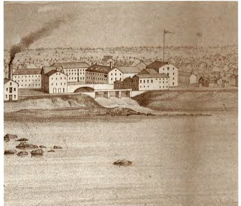
Edwin Whitefield's view of the Trenton riverfront in 1856 shows the embankment and aqueduct carrying the Trenton Water Power over the mouth of the Assunpink Creek. [Trenton Public Library]
