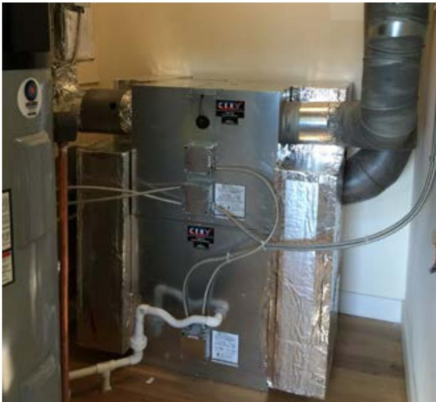
A Build Equinox Conditioning Energy Recovery Ventilator (CERV) is shown installed in the mechanicals room of a superinsulated 1,000-square-foot modular home in Vermont. The unit preconditions incoming air and delivers cooled or warmed fresh air to remote rooms as needed, controlling humidity and air quality as well as temperature.
