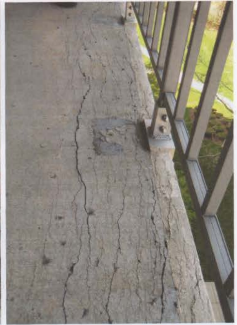
CRACKING CONCRETE Freeze-thaw cycling is a common cause of concrete deterioration where water infiltrates cracks, freezes and expands, causing a multitude of problems.
