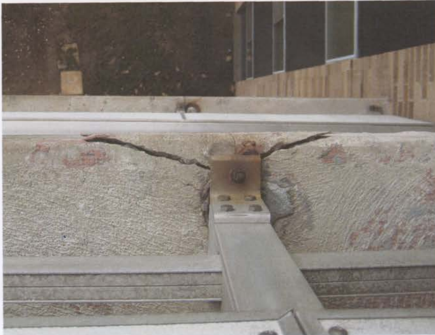
CRACKING CONCRETE Freeze-thaw cycling is a common cause of concrete deterioration where water infiltrates cracks, freezes and expands, causing a multitude of problems.
