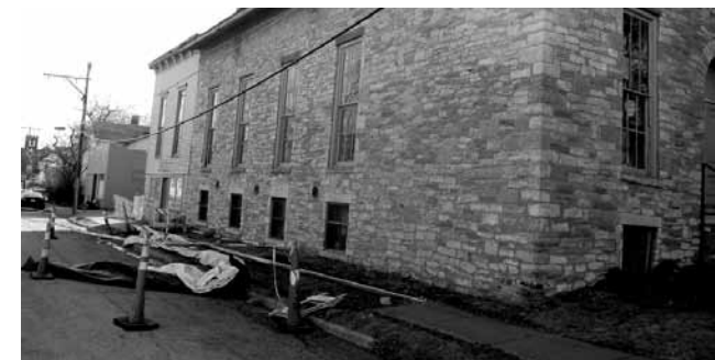
Replacement of a decrepit sidewalk is part of the Phase 1 rehab.
