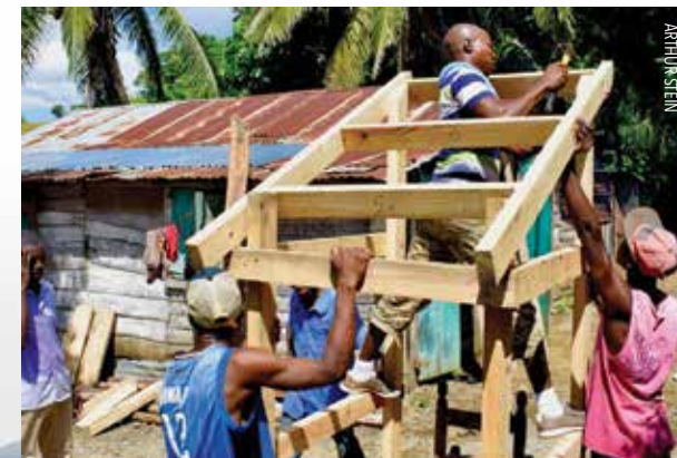
The building crew constructs houses for the latrines. These buildings offer privacy, as well as reduce the spread of disease by keeping flies away from the latrines.
