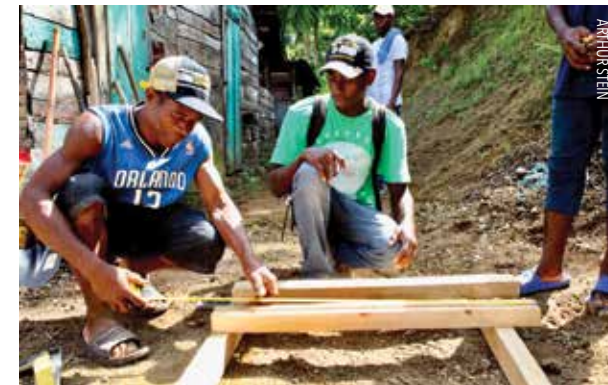
Members of the latrine building crew construct a mold for the latrine platforms.
