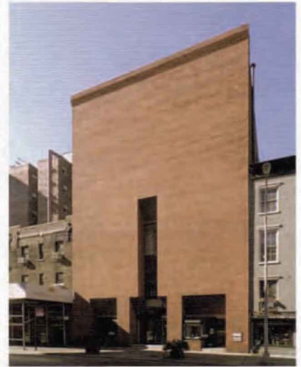
1966 FAÇADE, PRE-RESTORATION, CIRCA 2004
