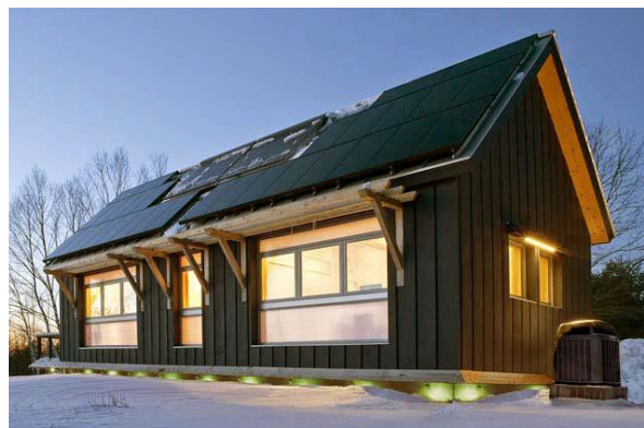
Figure 3. The BrightBuilt Barn by Kaplan Thompson Architects and Bensonwood Homes, Winner of the 2009 LEED for Homes Innovative Project Award
