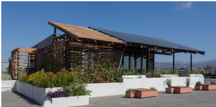
Figure 4. Arizona State University 2011 Solar Decathlon house. An example of “Legibility” and “Shading.”
