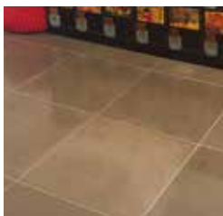
Concrete tiles and wall cladding
