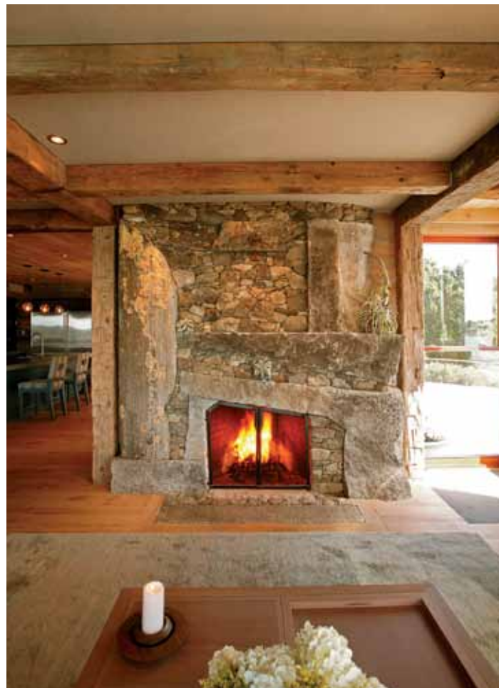
Master mason. Lew French is the craftsman behind all of the home's stonework. Using granite from old New England foundations and recycled fieldstone, Lew carefully selects and places each stone, rarely cutting or altering that rock. (For more on Lew and his work, see p. 106.)
