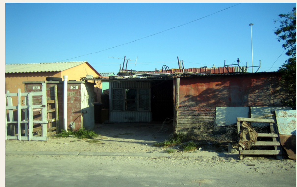
Khayelitsha Township, Western Cape Province
